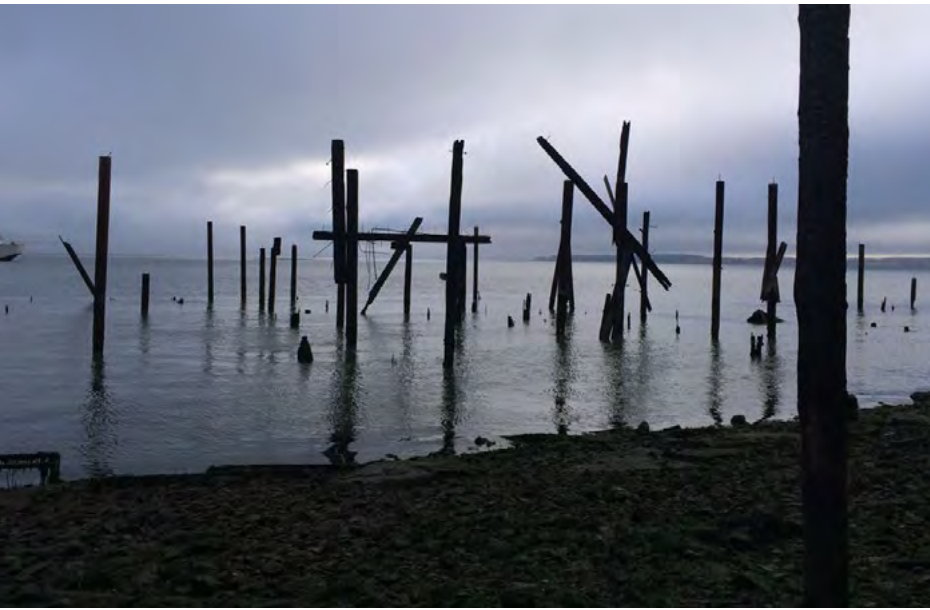
Creosote-treated pilings at the Red Rocks warehouse site in Richmond. Photo by Marilyn Latta, State Coastal Conservancy.
