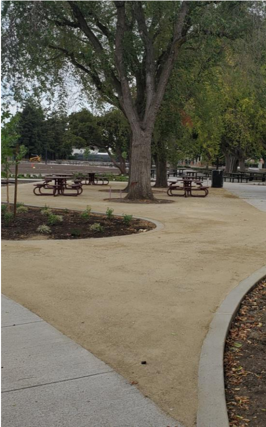
Decompose Granite (stabilized) pathways
