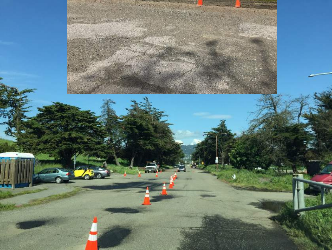
Street Improvement Projects at the Berkeley Marina Public Information Meeting – April 28, 2018
