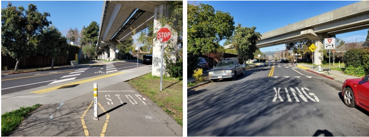
Existing conditions at Santa Fe Avenue crossing
