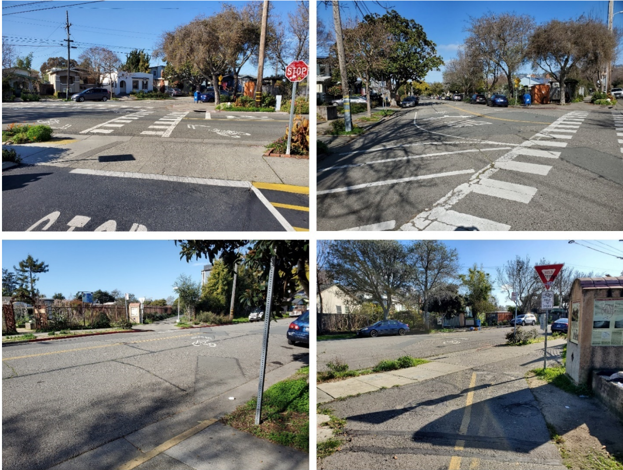
Existing conditions at Hopkins Street and Peralta Avenue crossing
