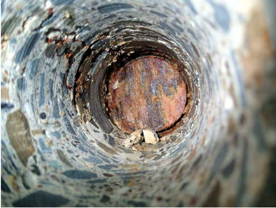
Photo 3-11: Inside view of concrete core showing timber pile
