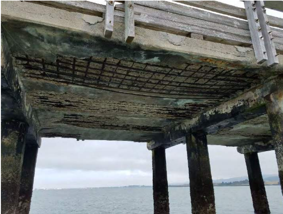
Photo 3-6: Typical Below Deck Condition of Section 2 Panels
