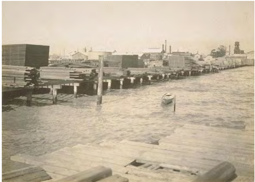
Photo 2-1: Original Pier Construction (Source: Bancroft Library, UC Berkeley)
