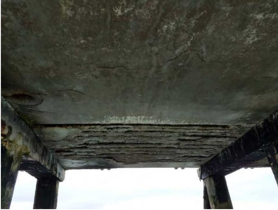
Photo 3-5: Typical Below Deck Condition of Section 1 Panels
