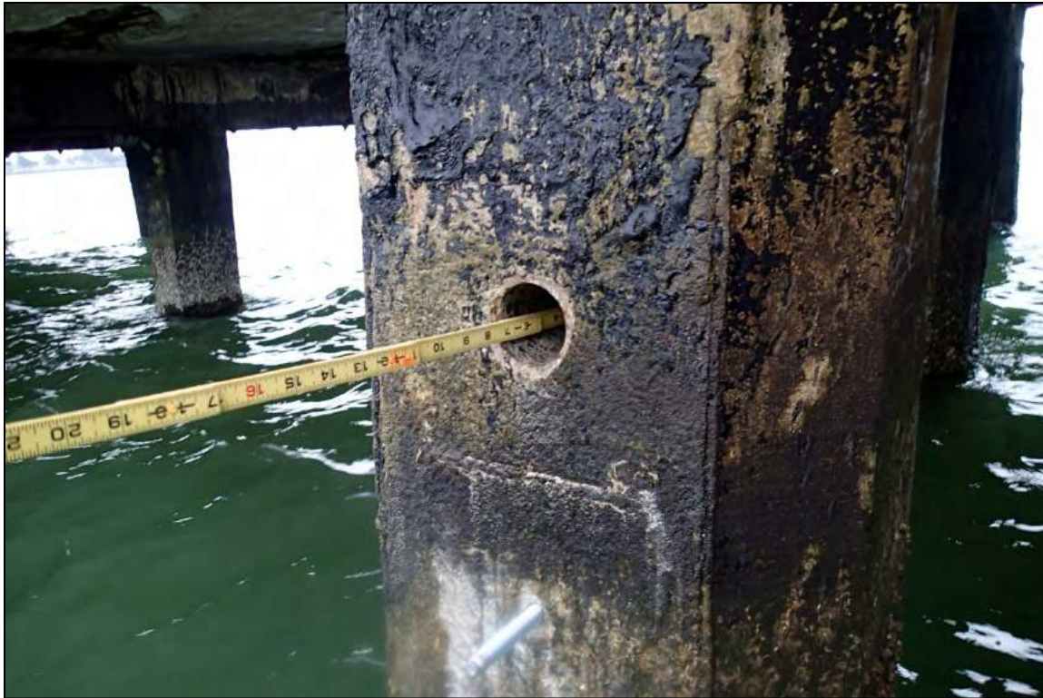
PHOTOGRAPH 21: Pile 429A, Level III concrete core hole
