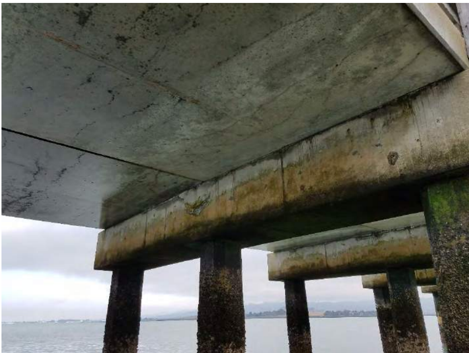
Photo 3-7: Typical Below Deck Condition of Section 3 Panels
