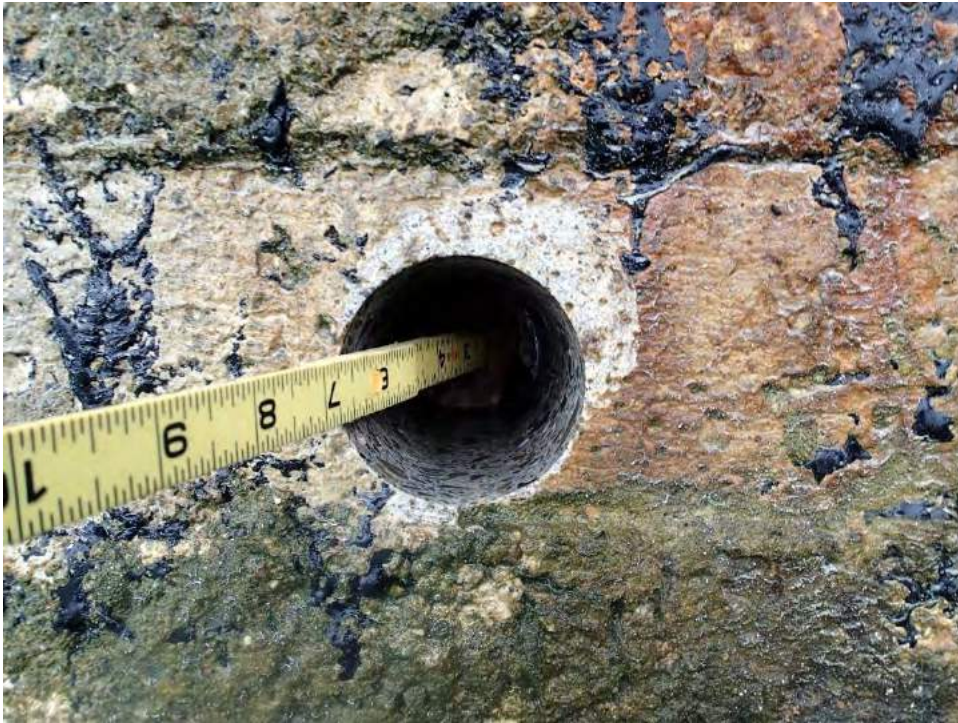
Photo 3-10: Core of concrete pile jacket
