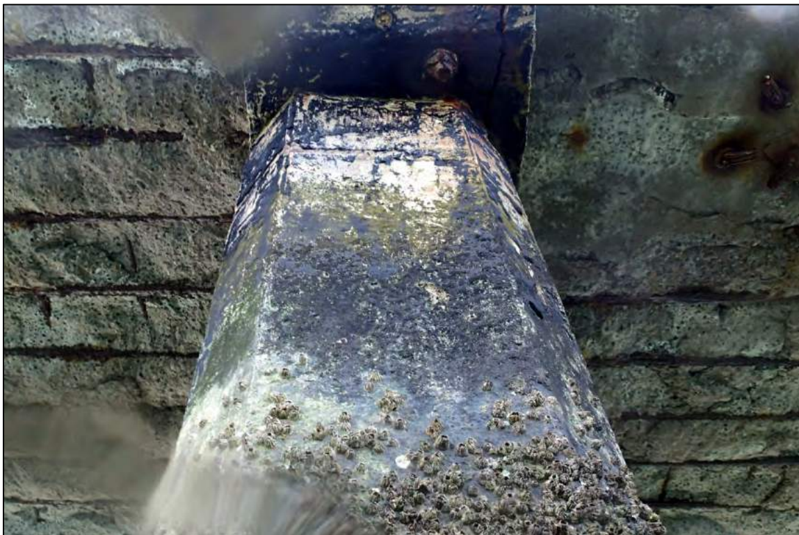
PHOTOGRAPH 20: Pile 366A, undamaged
