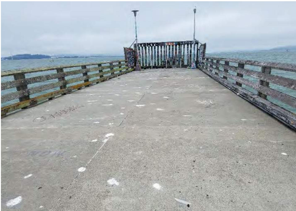
Photo 3-4: Typical Above Deck Condition of Section 3 Panels
