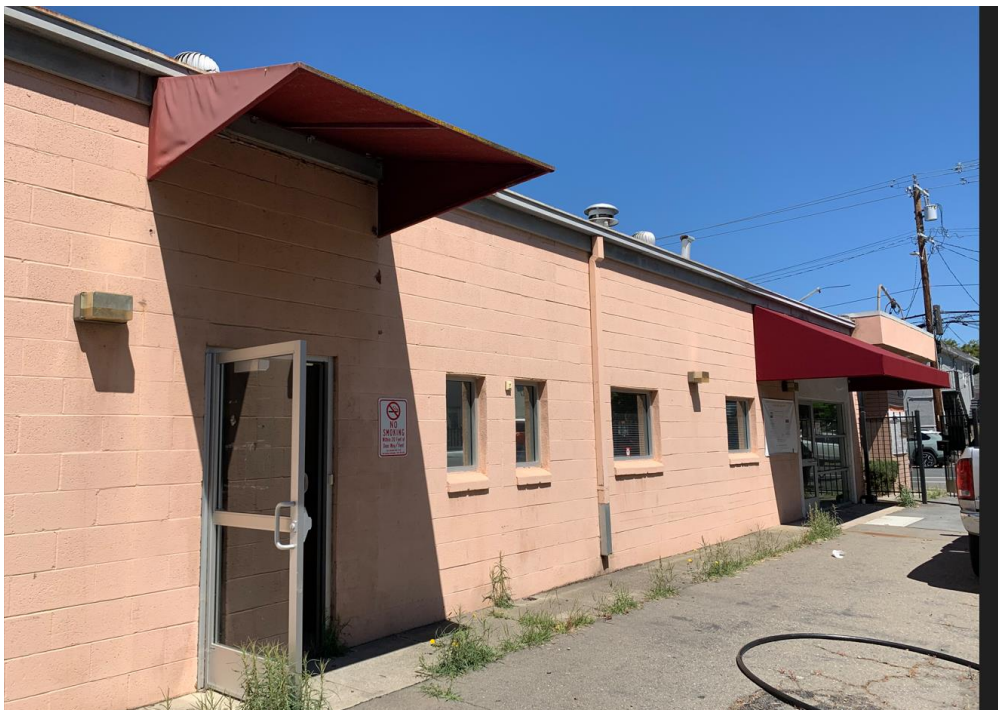
Figure 8. Exterior East Wall
