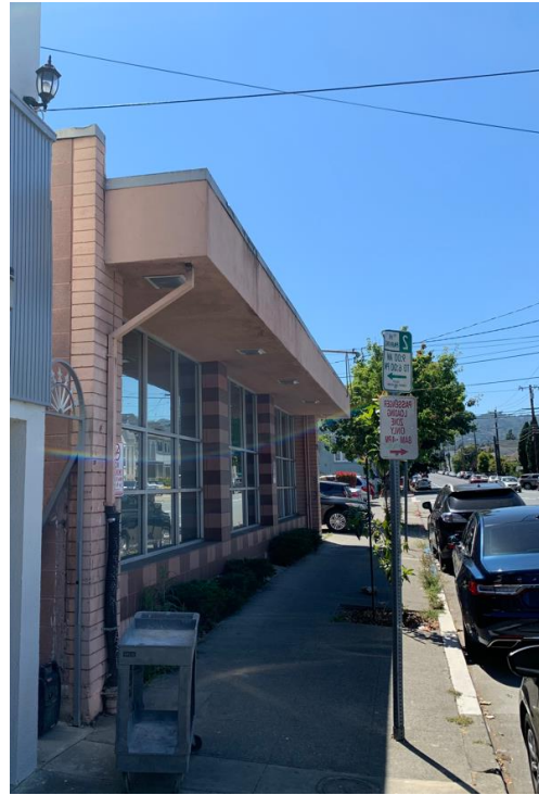
Figure 10. View looking at Front
