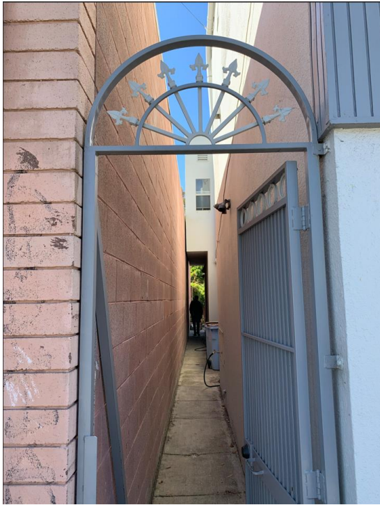
Figure 9. Exterior West Wall
