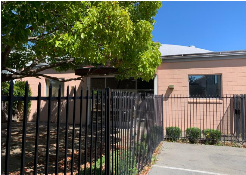
Figure 11. Exterior South Wall
