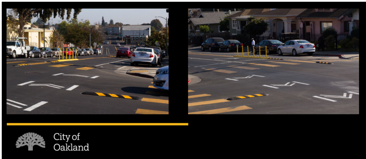
“Hardened Centerline” with flex posts and speed bumps for left turn hardening
