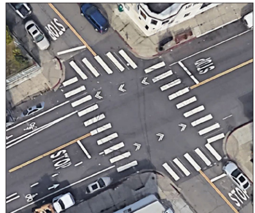
Figure 3: Intersection chevron markings, 38th Ave and Brookdale Ave
