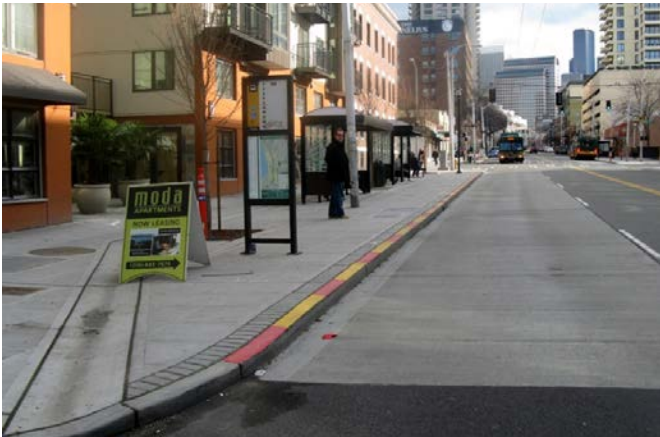
Figure 3.5. Bus Pad in Seattle, Washington. (Source: NACTO, B. Bryant)
