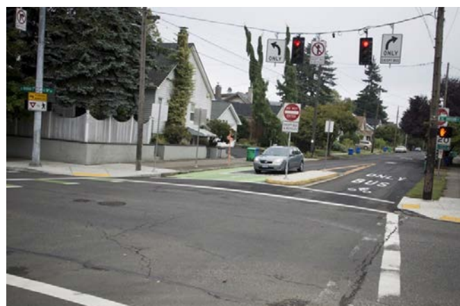
Figure 3.16. Transit-only Aperture in Portland, Oregon. (Source: PBOT)
