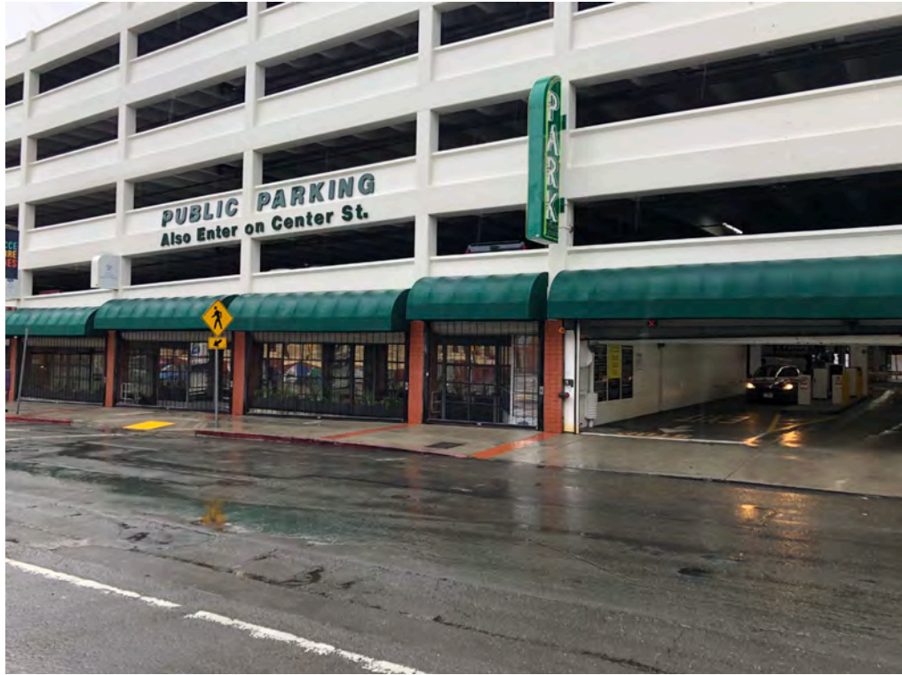
Photograph 6: Public parking garage, looking northwest.
