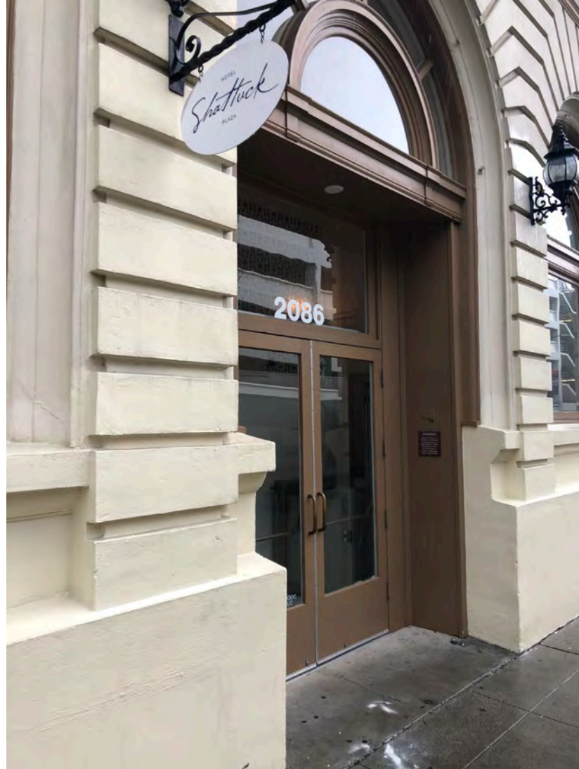
Photograph 5: Hotel Shattuck, looking southwest.
