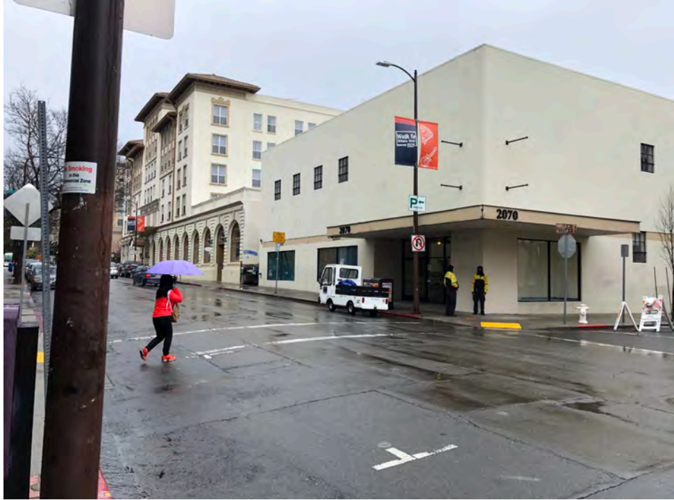
Photograph 1: Site building, looking southeast.
