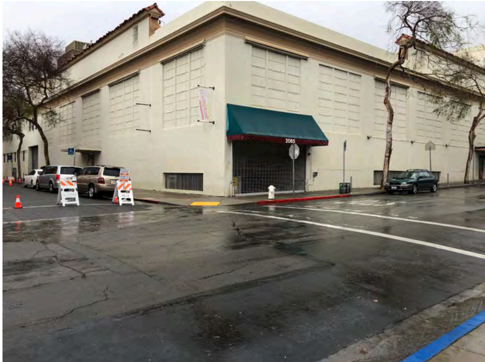
Photograph 2: West side of Site building, looking southeast.
