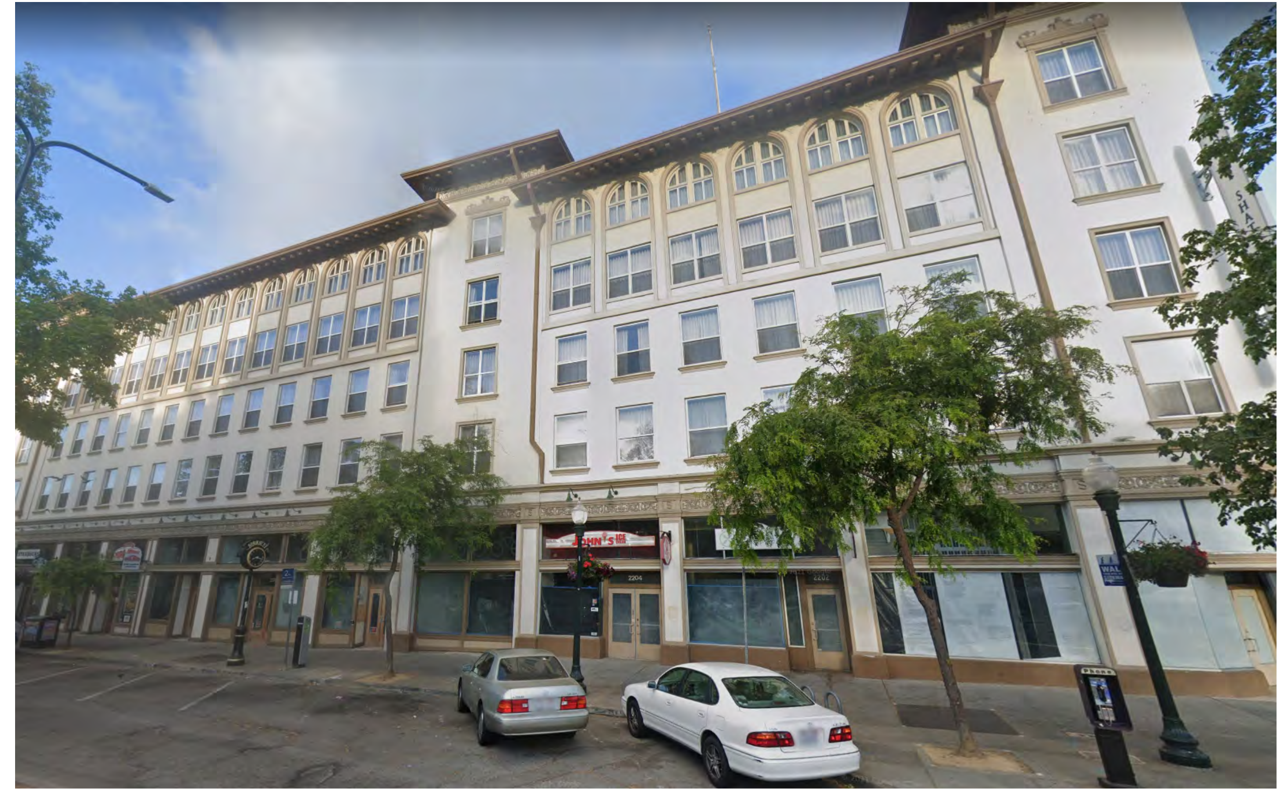
2 SITE PHOTO - SHATTUCK AVE - EXISTING HOTEL A0-003 12" = 1'-0"
