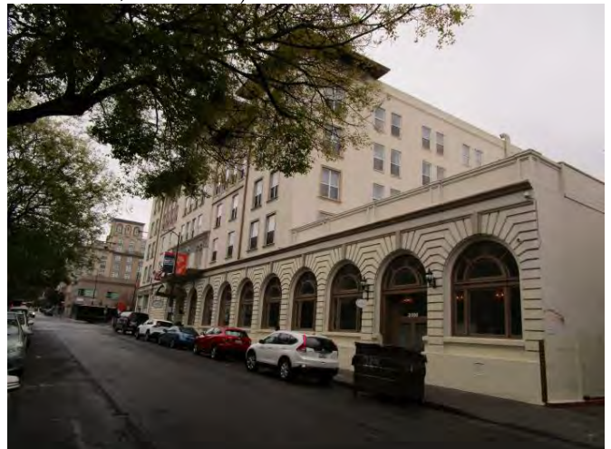
North elevation, view southeast. (Rincon Consultants, March 2022).
