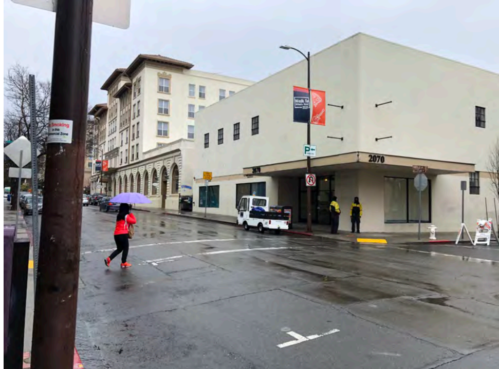
Photograph 1: Site building, looking southeast.
