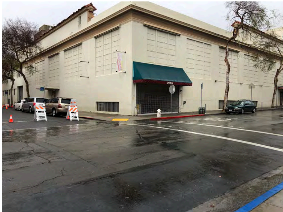
Photograph 2: West side of Site building, looking southeast.
