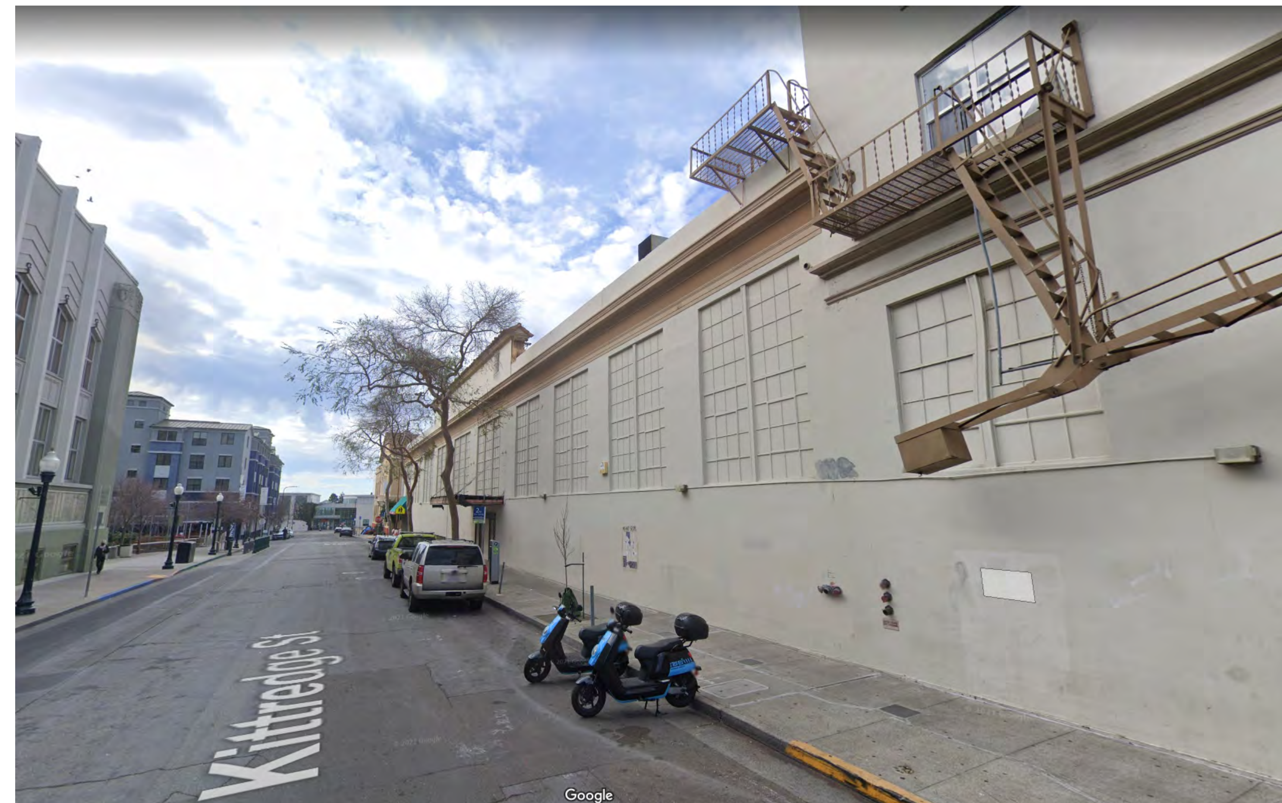
4 SITE PHOTO - KITTREDGE ST - LOOKING WEST A0-001 12" = 1'-0"
