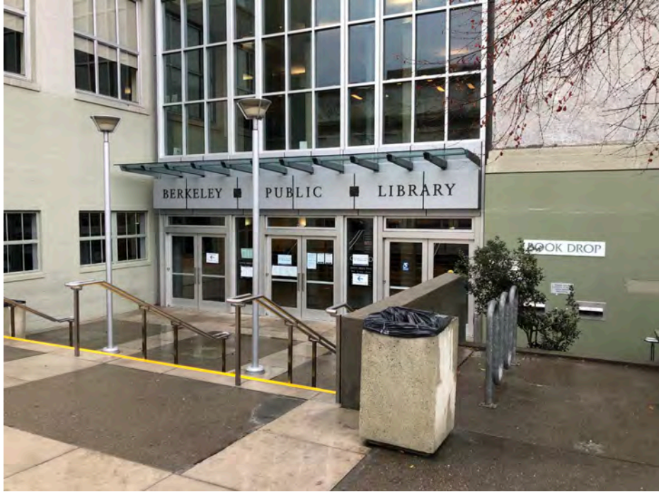
Photograph 3: Berkeley Public Library, looking southeast.
