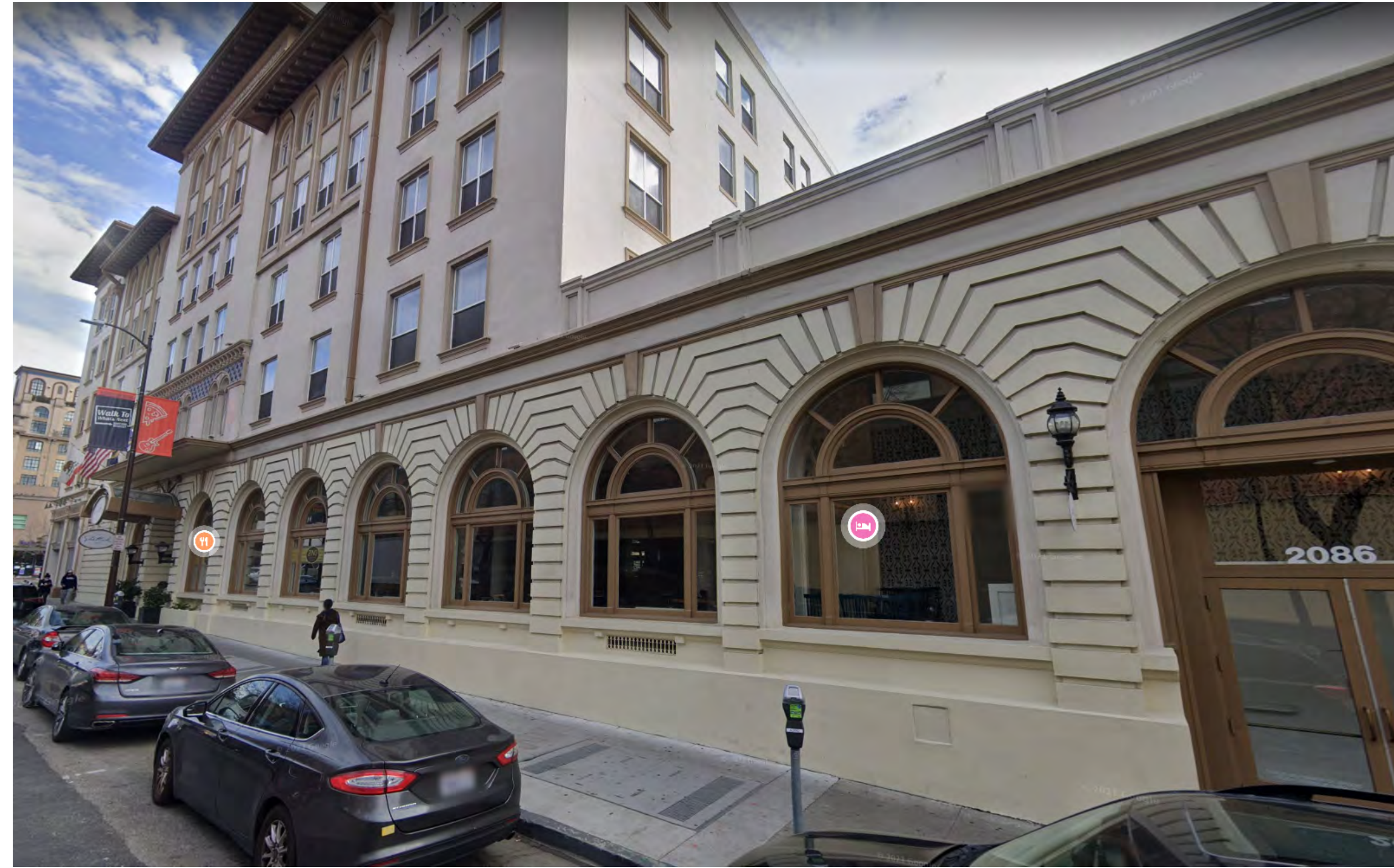
1 SITE PHOTO - ALLSTON WAY - EXISTING HOTEL A0-003 12" = 1'-0"
