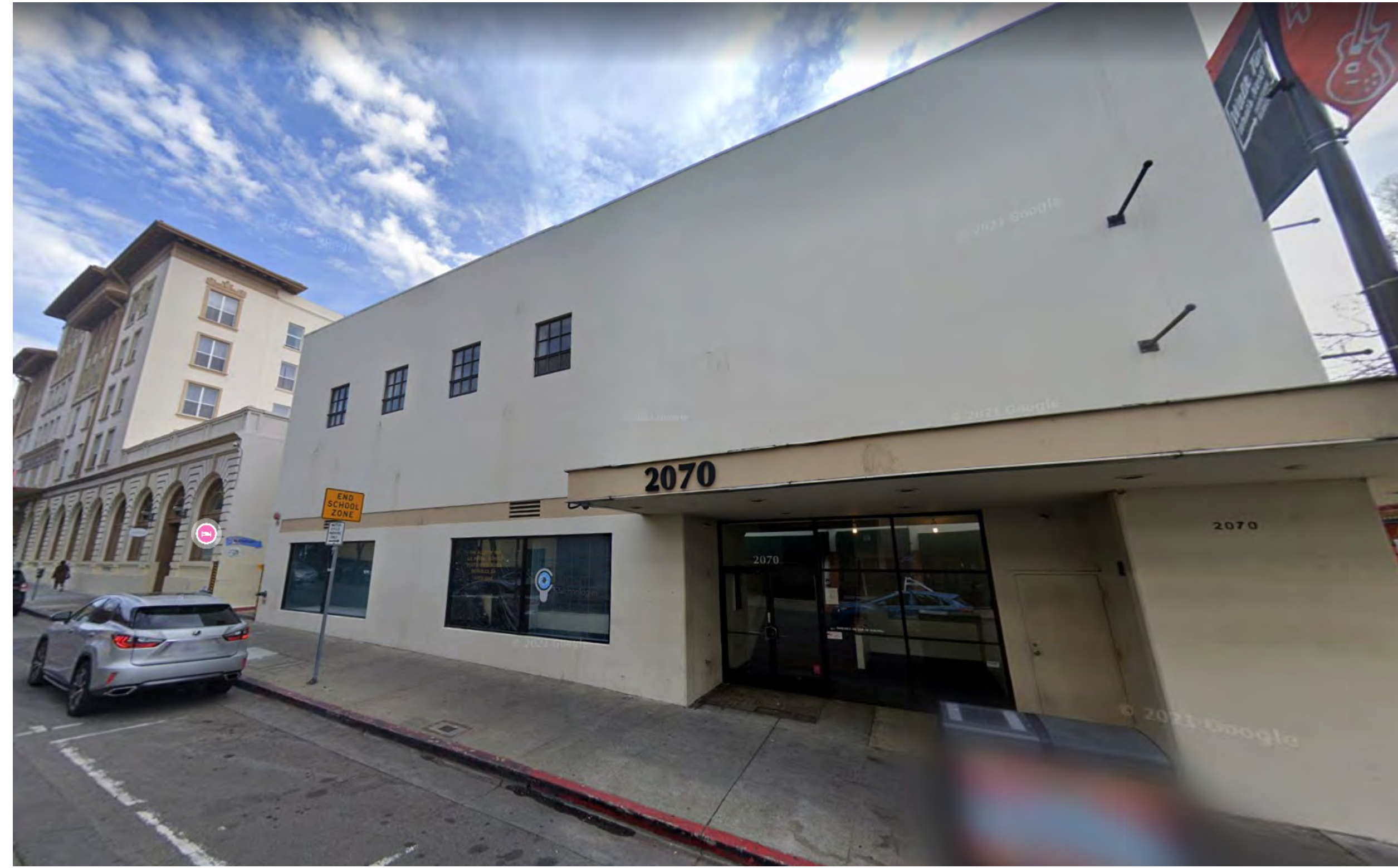
1 SITE PHOTO - ALLSTON WAY FACADE A0-002 12" = 1'-0"
