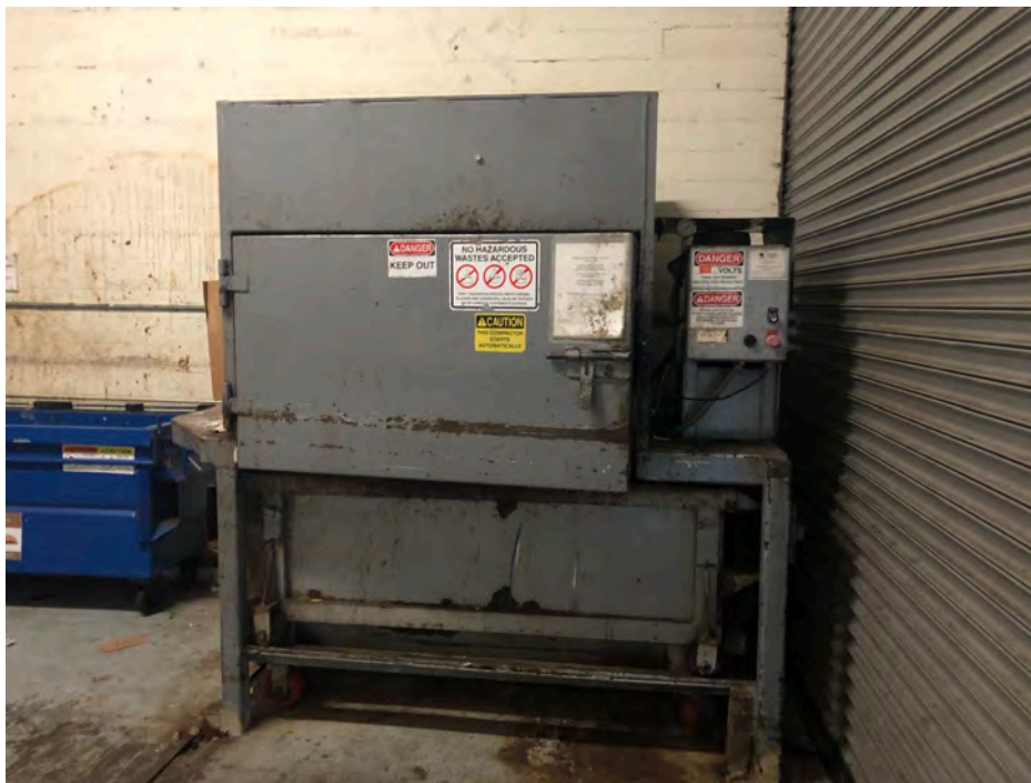
Photograph 10: Trash compactor, looking south.
