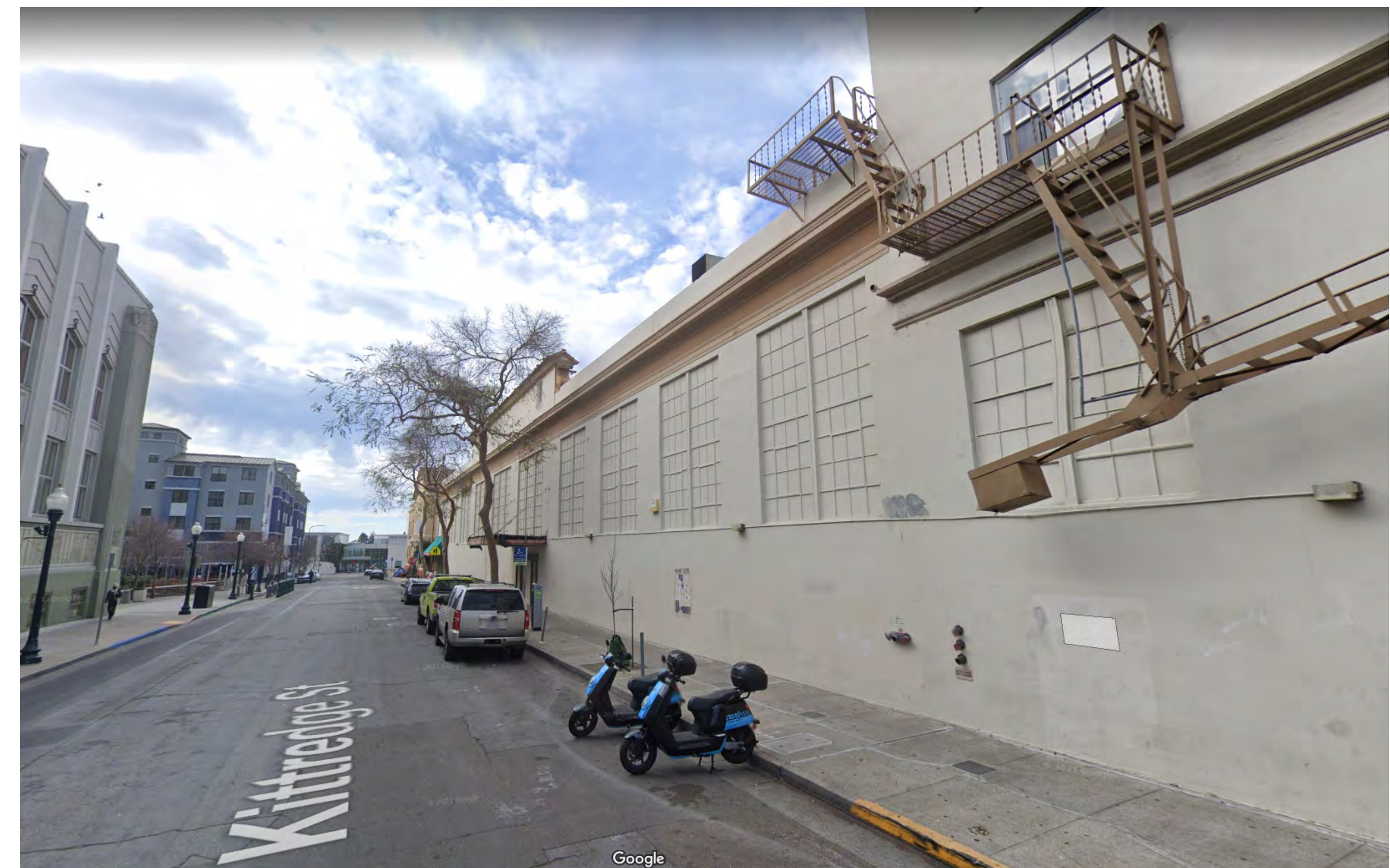
4 SITE PHOTO - KITTREDGE ST - LOOKING WEST A0-001 12" = 1'-0"
