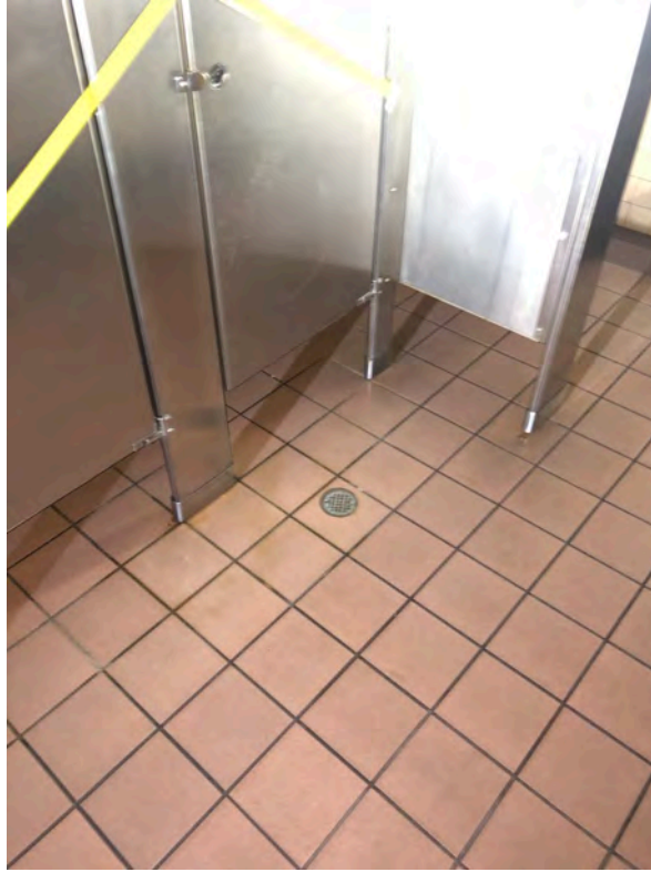
Photograph 12: Bathroom floor drain.
