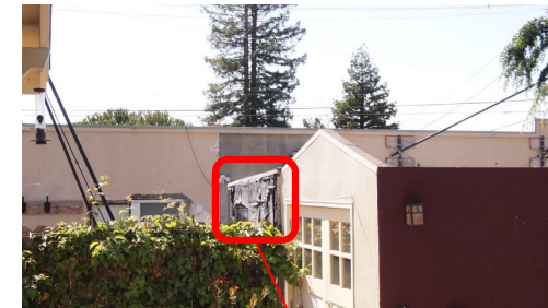
Current shed barely visible over fence
