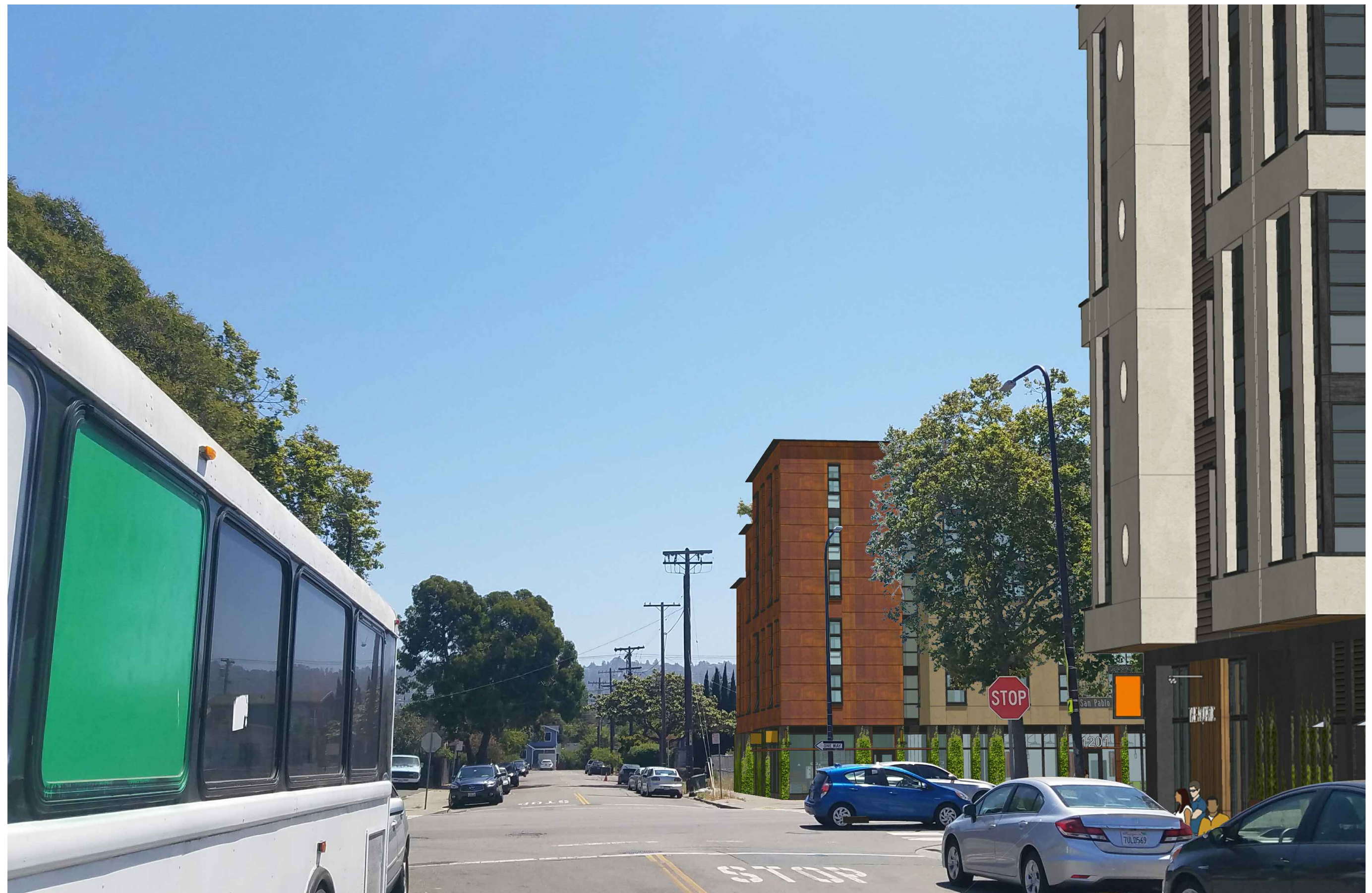
4 HARRISON LOOKING EAST - AFTER
