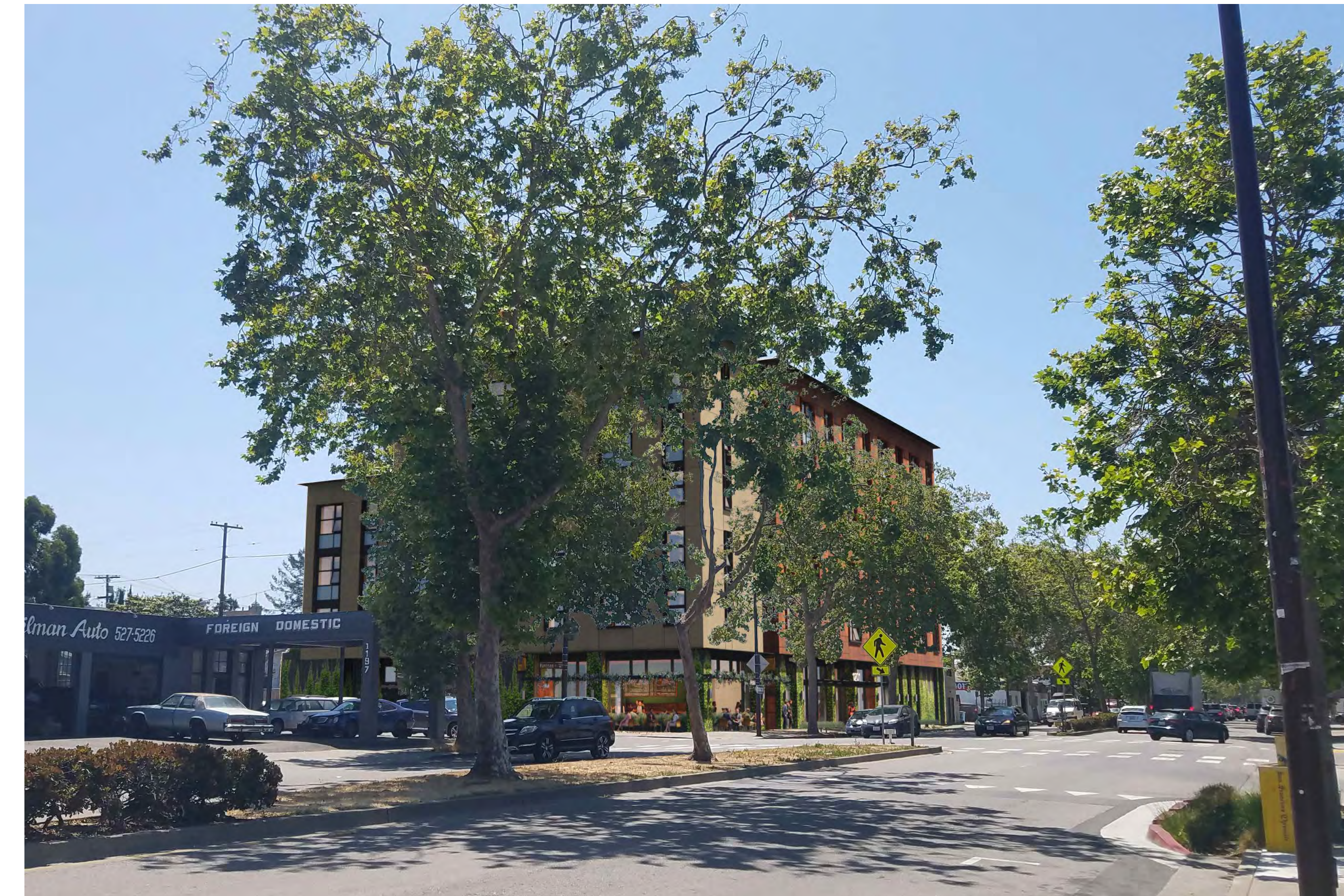
2 SAN PABLO LOOKING SOUTH - AFTER
