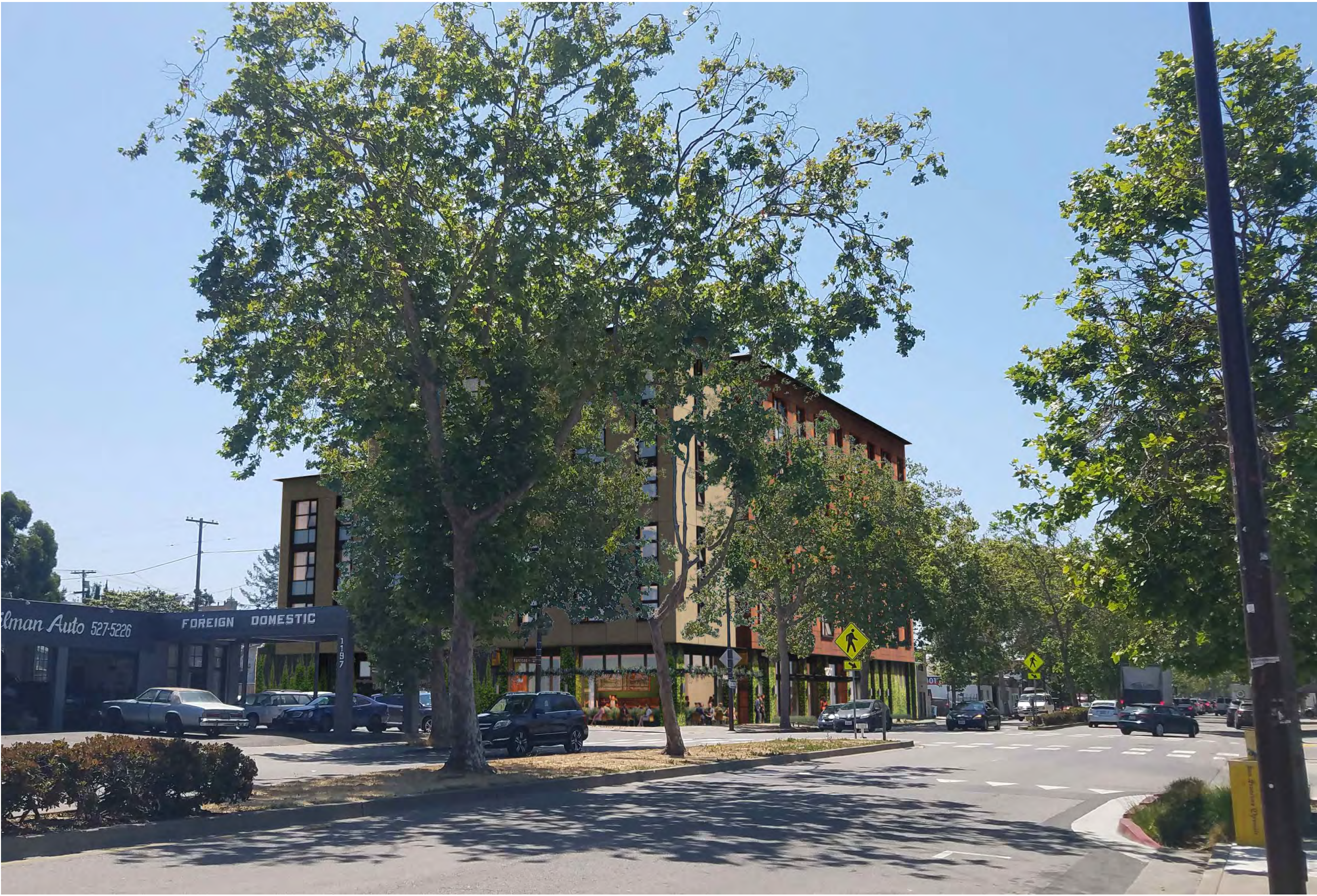
2 SAN PABLO LOOKING SOUTH - AFTER
