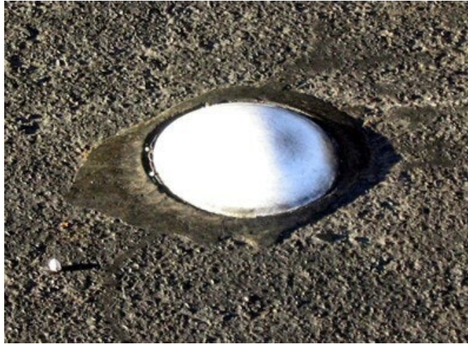
Close up of bott's dot.
