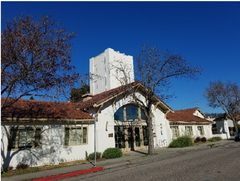
Fire Training Building, Berkeley
