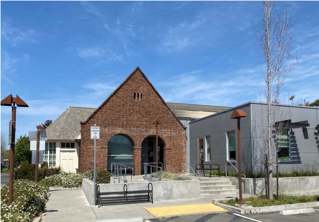
Corporation Yard Building
