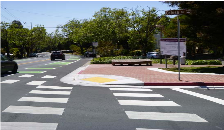
Curb ramp on Colusa Avenue
