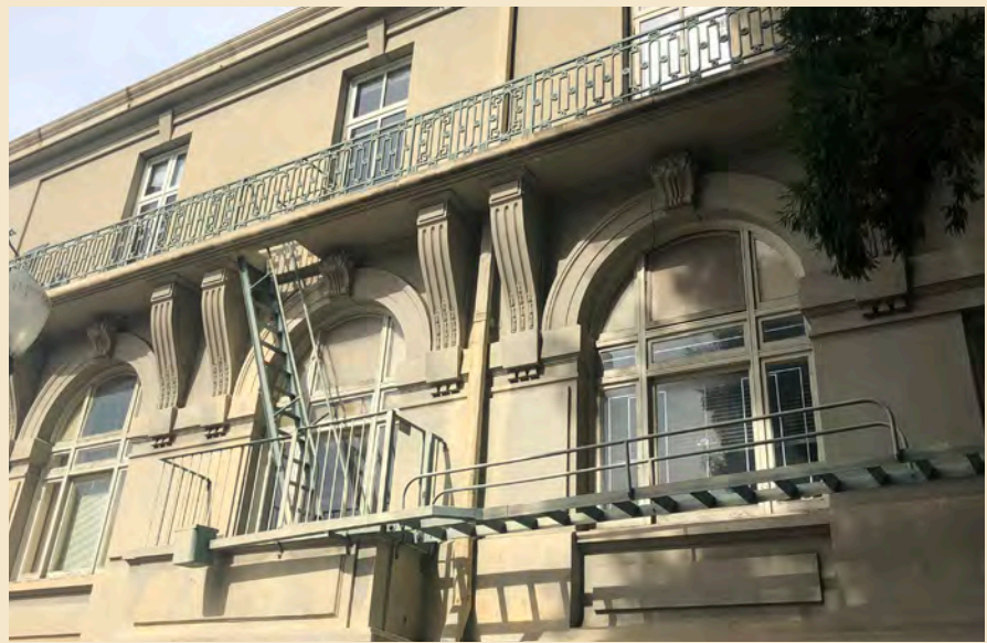
Figure 6.11 First floor balcony and modern metal fire escape at south (side) façade.
