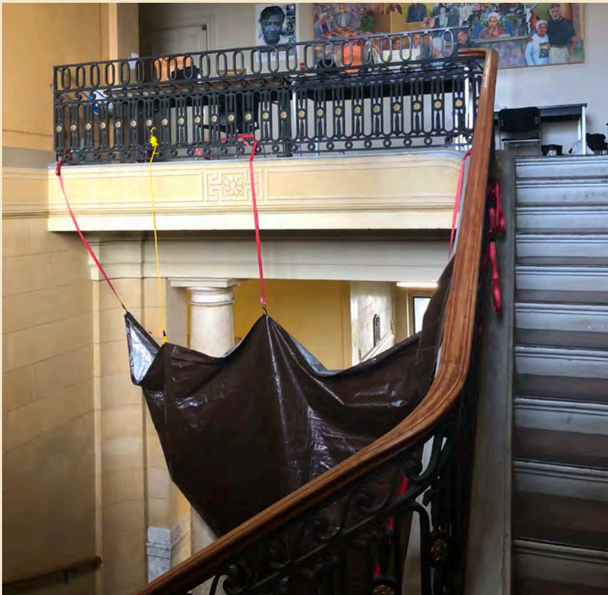
Figure 7.16 The double height space with stairs below at the main staircase will make access to the ceiling and original pendant light fixture difficult.
