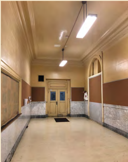
Figure 6.20 Rectangular fluorescent light fixtures in main corridor.
