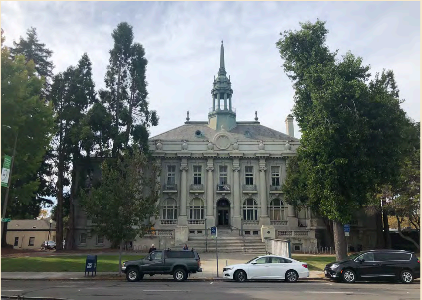
Figure 6.5 East (front) façade.
