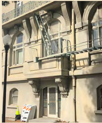
Figure 6.17 Balcony with a solid paneled balustrade at south (side) façade.
