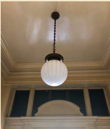
Figure 6.23 Original pendant light fixture in the entry vestibule.
