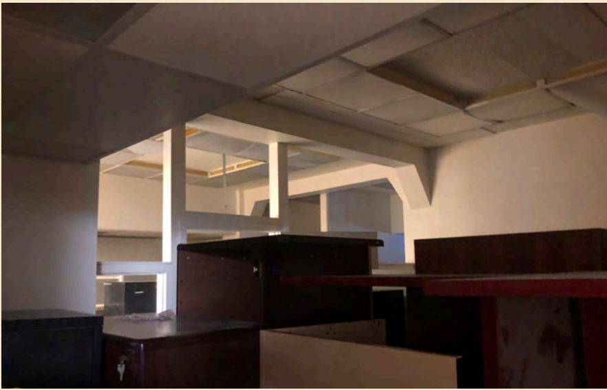
Figure 6.29 Original structural columns and beams in the basement.
