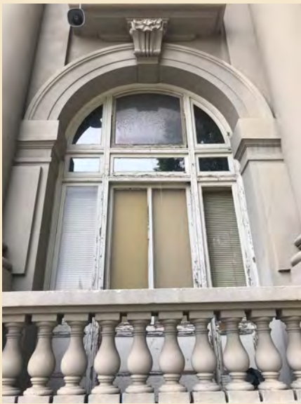
Figure 6.15 Semicircular-arched window with pronounced springers and ancon and swag keystones are found throughout the building.
