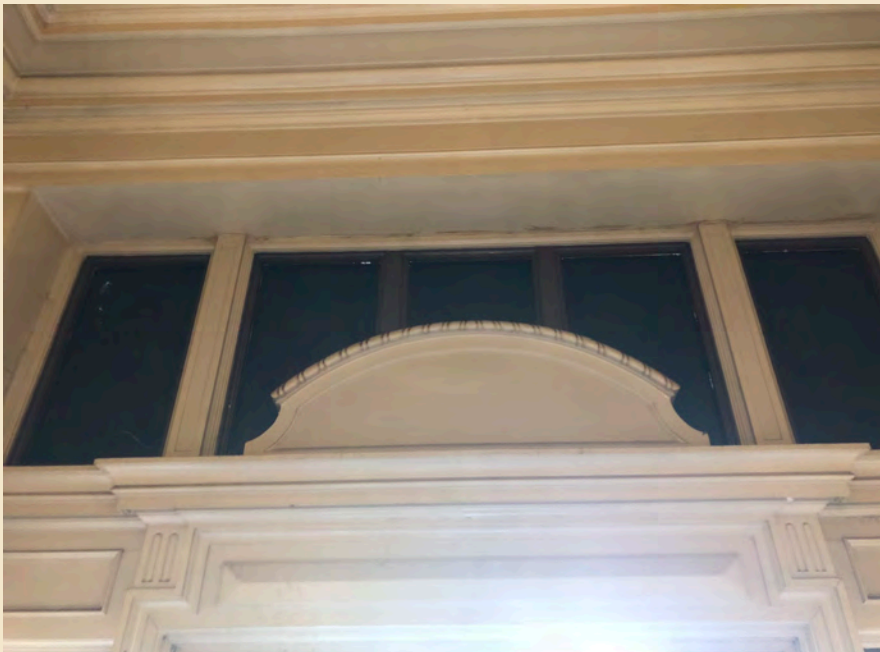
Figure 7.10 The transom of the building's primary (east) entry has been back painted.
