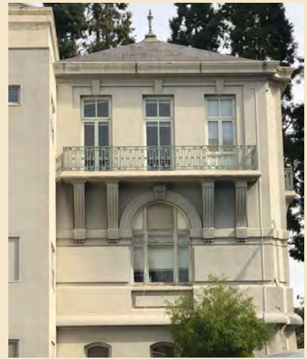
Figure 6.18 Original nine-part windows at west (rear) façade.
