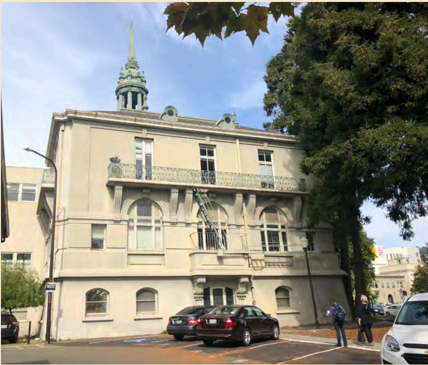
Figure 6.10 South (side) façade.
