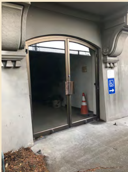
Figure 6.12 Entrance at north (side) facade.
