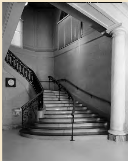
Figure 6.21 1981 HABS photograph of the Main Stair.
