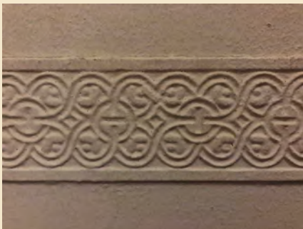
Figure 6.26 Remnant plaster chair rail in the south wing.
