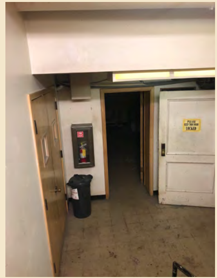
Figure 6.30 Remnant paneled wood door in basement.
