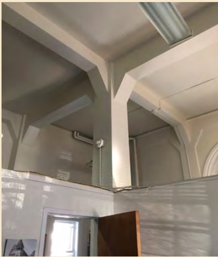
Figure 6.25 Original structural columns and angled elements where they meet the ceiling in first floor of the south wing.
