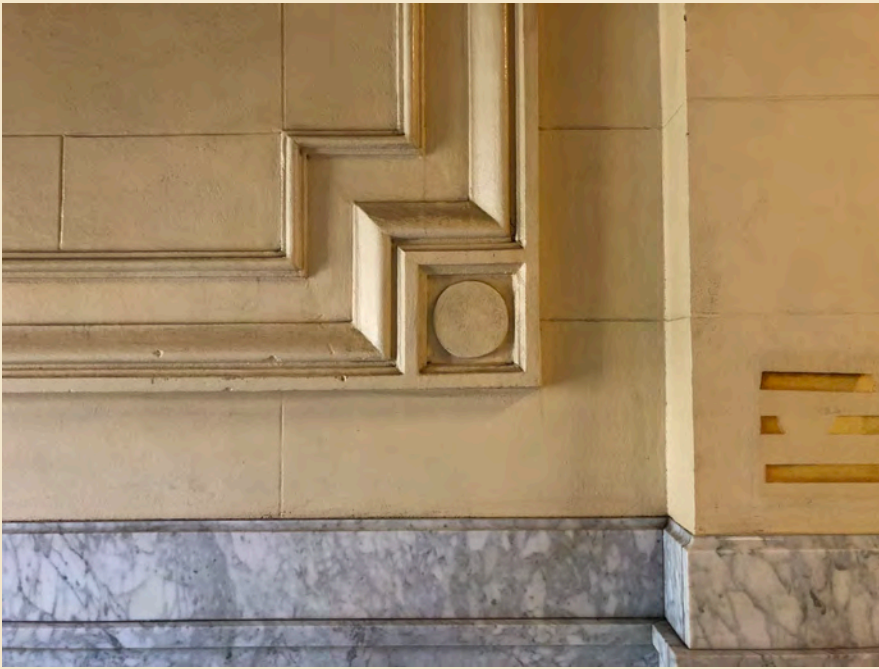
Figure 6.19 Light grey marble dado and wide bands of plaster moulding forming decorative panels in the entry vestibule.
