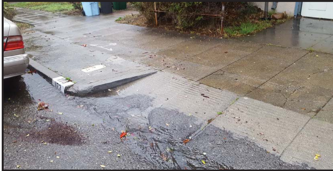
Figure 1: Water Flow at Project Site Frontage (1173 Hearst looking southwest)
