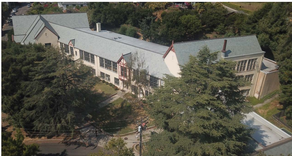
Figure 3 : Partial Aerial photograph of subject building, looking northeast
