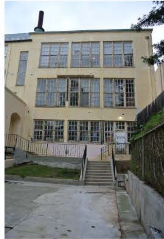
SOUTH ELEVATION PHOTO
