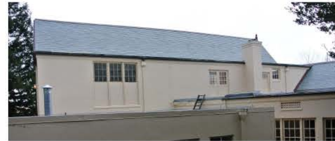
NORTH ELEVATION PHOTO
