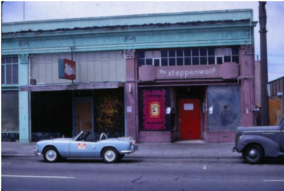
Borg Building, 1967, Humphrey Slide Collection, BAHA
