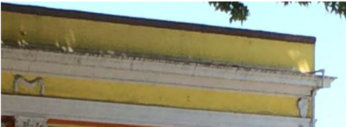
Architrave and Parapet, Borg Building, 2020, Fran Cappelletti
