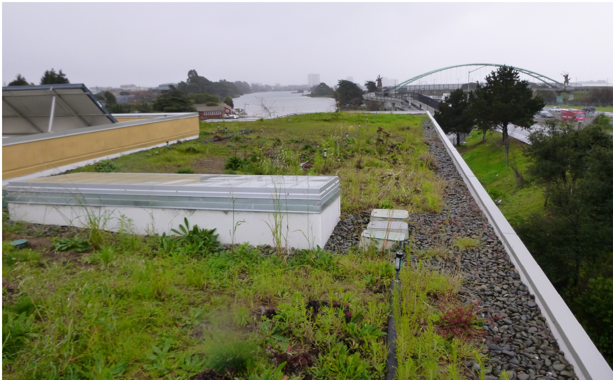
Figure 8 – The green roof at the City of Berkeley's Dona Spring Animal Shelter.
