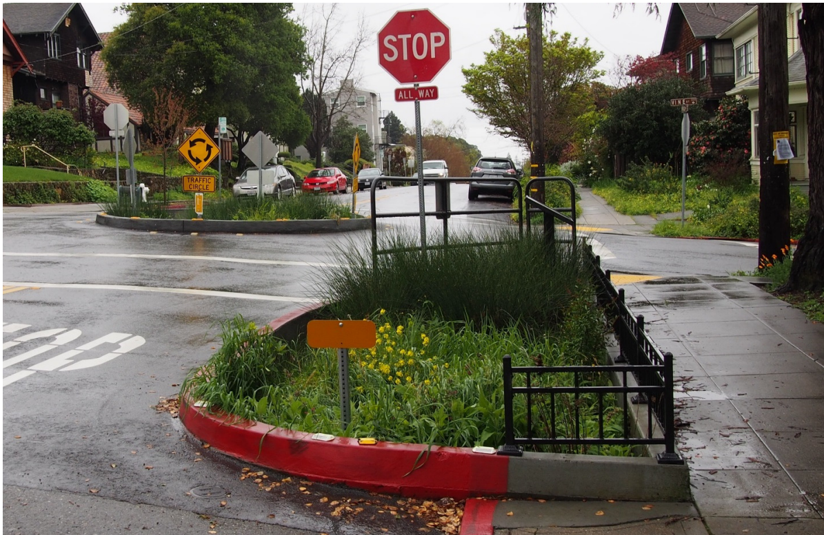
Figure 7 – Connected bioretention features in a traffic circle and corner bulb-out at Spruce and Vine Streets.
