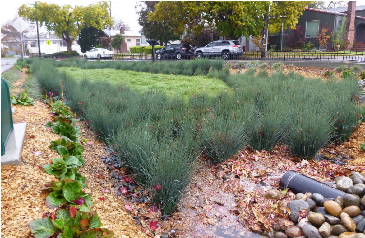
Figure 5 – A large concrete traffic island/median was reconstructed with a bioretention facility at Rose and Hopkins Streets.
