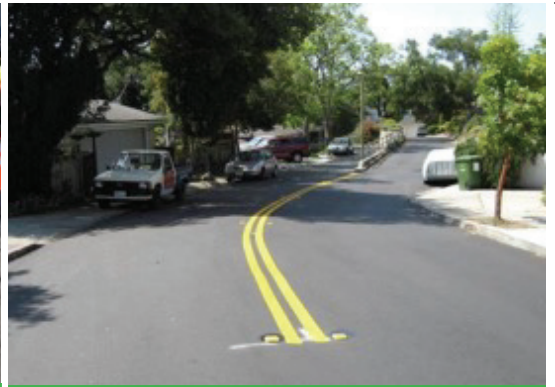
Completed street surface overlay
