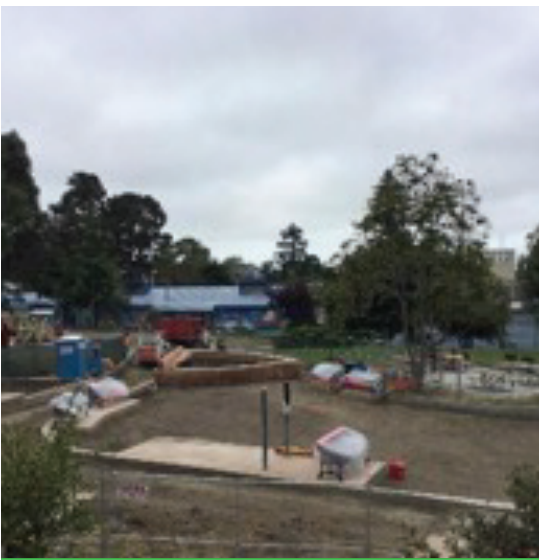
King Park renovation
