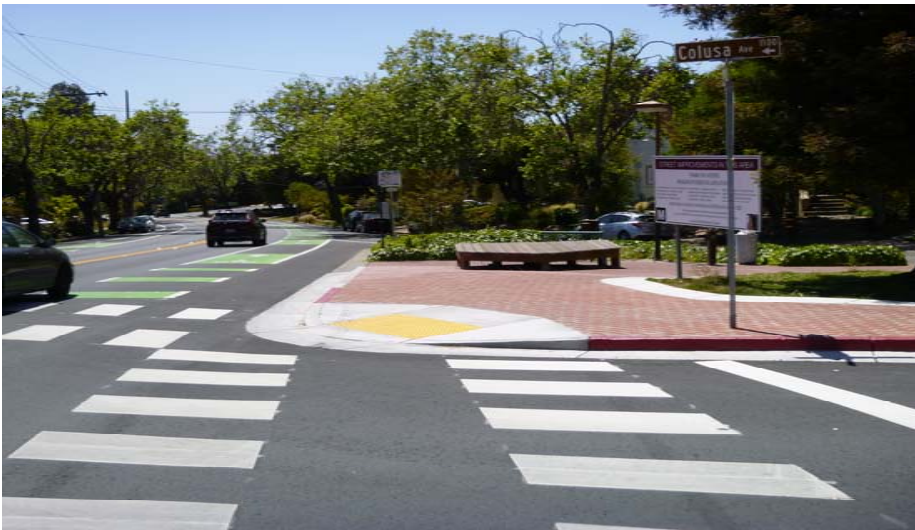
Curb ramp on Colusa Avenue
