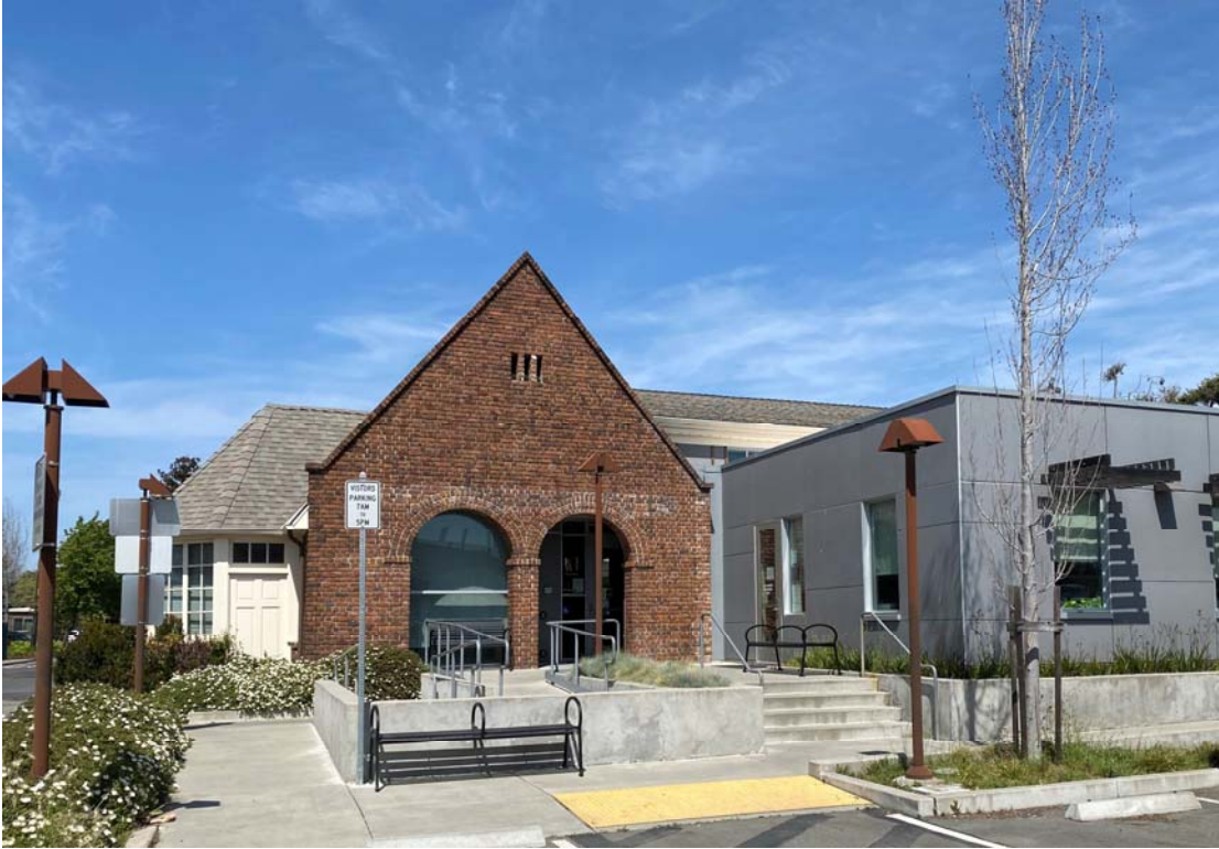
Corporation Yard Building
