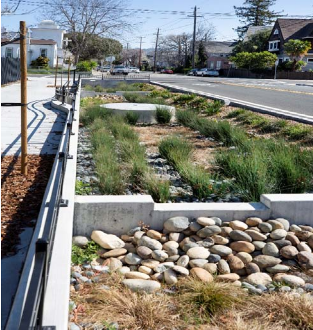
Green infrastructure installation at Woolsey Street
