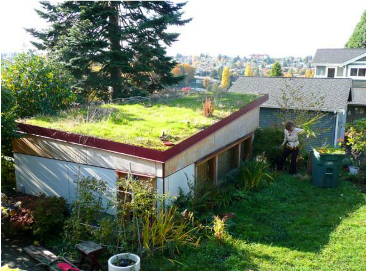
Figure 3-5, Garage Green Roof in Mount Baker
