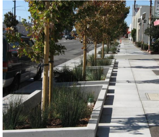
Figure 3-11, El Cerrito Rain Garden Project, San Pablo Ave.
