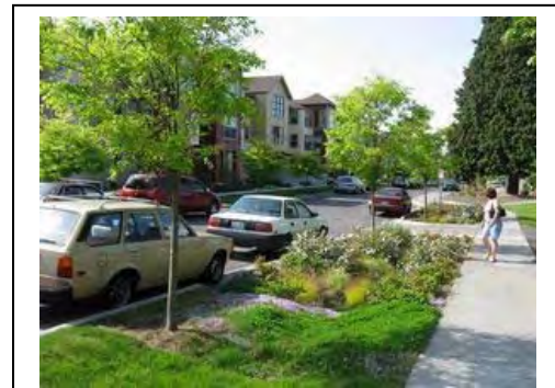
Bioswales serve to filter pollutants from stormwater and reduce peak surface runoff. This installation of these types of GI improvements would improve water quality.
