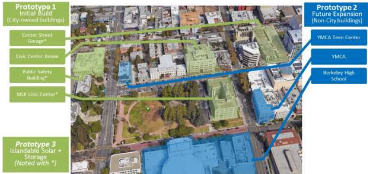
Figure 1: Berkeley Energy Assurance Transformation Building Locations
