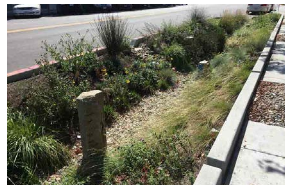
Curbside stormwater retention
