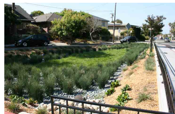
Integrated stormwater retention and sidewalk
