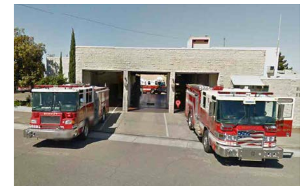
Berkeley Fire Station Number 5 on Adeline Street at Derby
