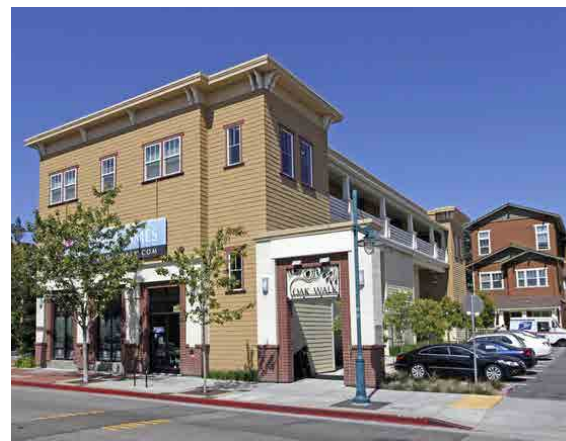
Parking lot located behind building
