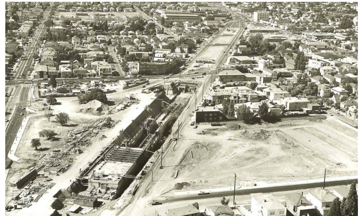
BART Construction at Ashby Avenue, circa 1967
