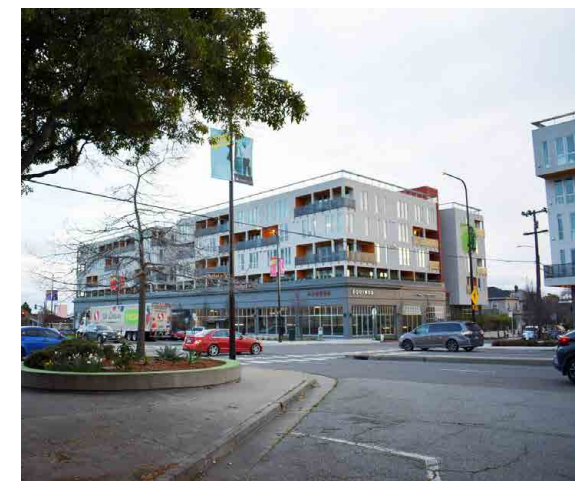
Existing mixed-use building in the South Shattuck subarea
