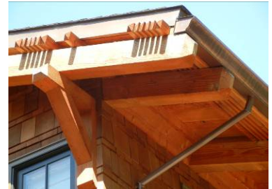
Building with copper flashing, gutter and drainpipe.
