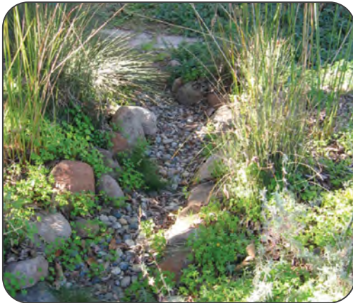
Dry creek infiltrates and conveys runoff.
