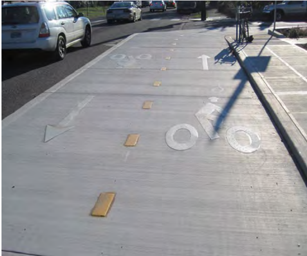
Pavement markings provide clear delineation between bi-directional bicycle traffic
