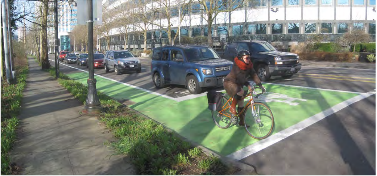
A bike box allows for cyclists to wait in front of queuing traffic, providing high visibility and a head start over motor vehicle traffic.
