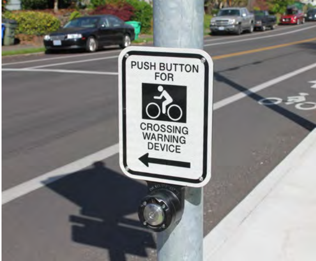
Bicycle push button actuators are positioned to allow bicycle riders in roadway to stop traffic on busy cross-streets.
