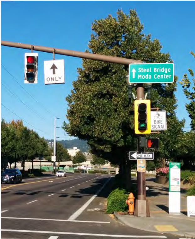
Bicyclists receive a green bike signal indication in advance of adjacent travel lane
