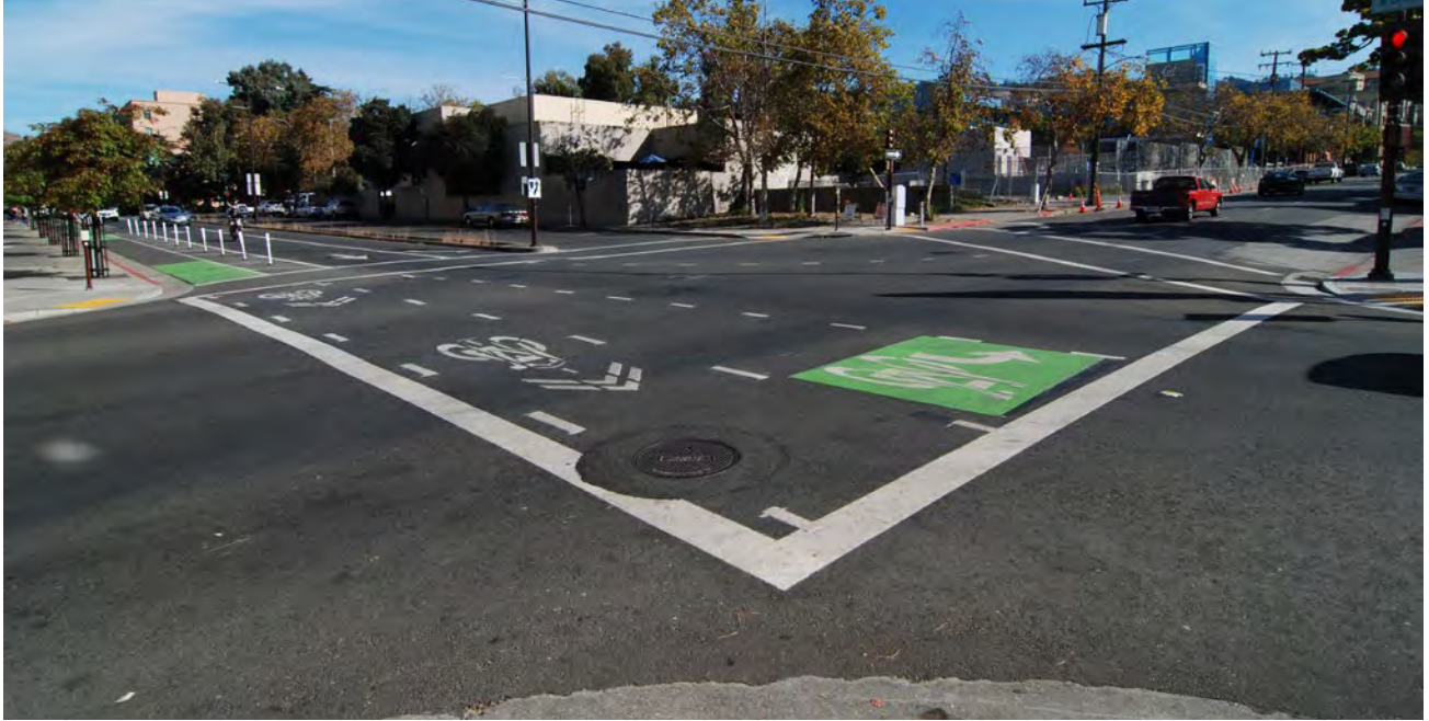
On separated bike lanes, the two-stage turn box can be located in the protected buffer/parking area.
