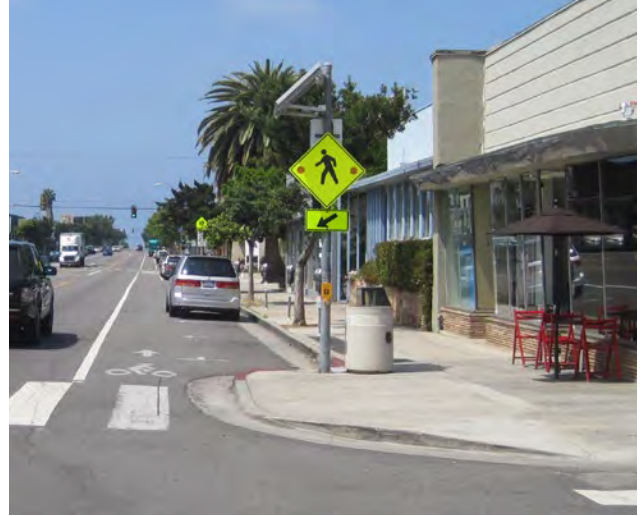
Curb extensions can be located at intersections or mid-block locations with an existing parking lane. This creates a de facto parking setback from the curb which increases visibility of pedestrians and bicyclists crossing the street.
