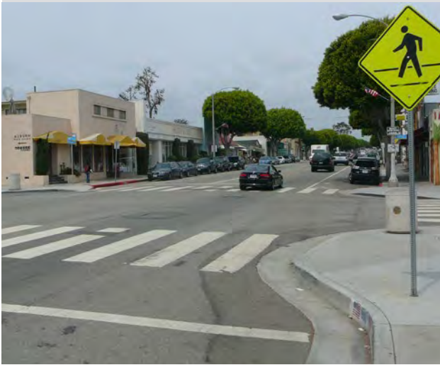
Curb extensions help to shorten the pedestrian crossing distance and visually narrow the roadway.
