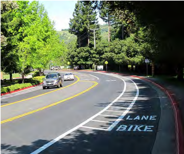
The use of pavement markings delineates space for cyclists to ride in a comfortable facility.
