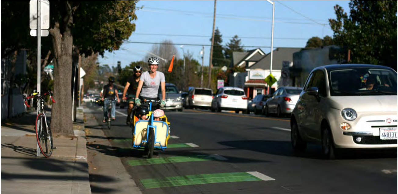
A colored bicycle lane on Laurel Street in Santa Cruz, CA alerts users to potential merging in advance of an intersection. Photo by Richard Masoner via Flickr (CC BY-SA 2.0).
