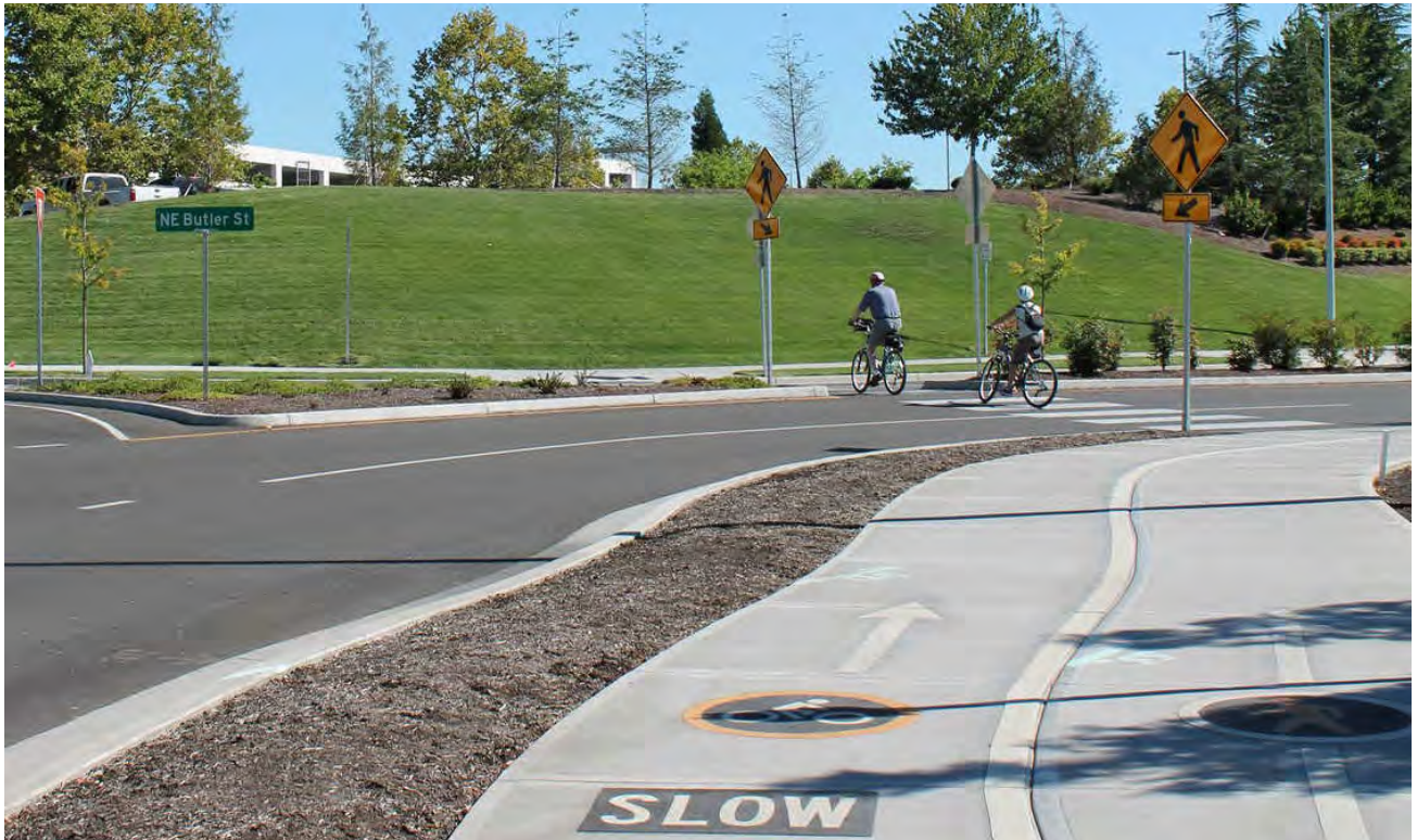
This roundabout with a separated bikeway and sidewalk help reduce conflicts between motorists and bicycle riders.
