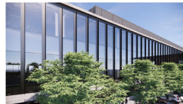
2: Inner West facade solid metal panels and decorative fins
