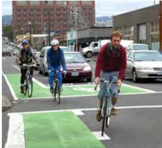
Figure f.7. Bike Boxes. Bike boxes put bicyclists in front of motor vehicles at intersections. Bike boxes improve bike safety and can enhance a street's overall performance.
