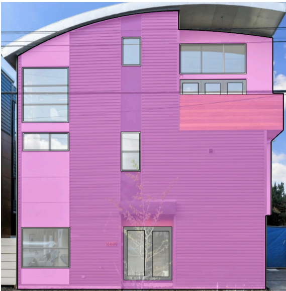
1444 Fifth Street, Berkeley Openings are approximately 19%
