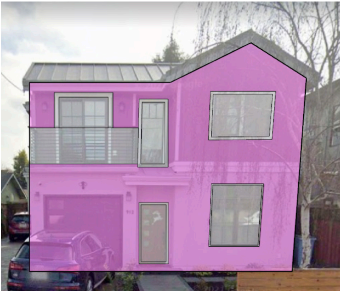
908 Cedar, Berkeley Openings are approximately 30%
