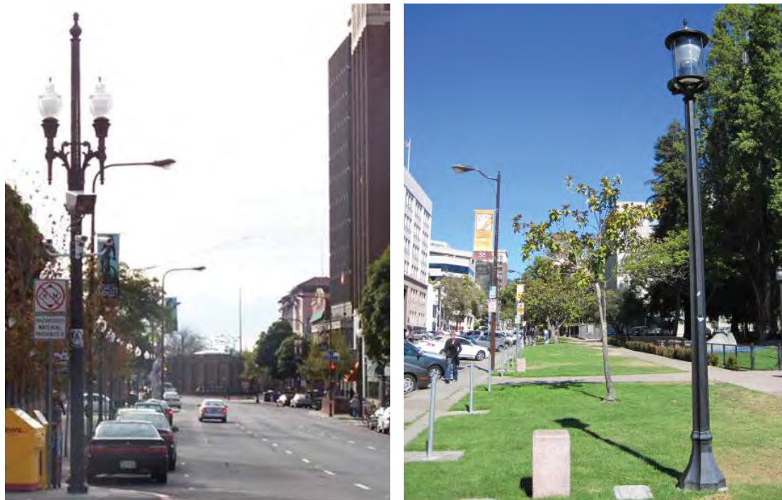
Figure 1.3. Traditional Light Fixtures. Traditional “acorn” light fixtures are extensively used and complement Downtown’s historic resources (left). To accentuate the Civic Center Historic District, different historic light fixtures were selected (right).
