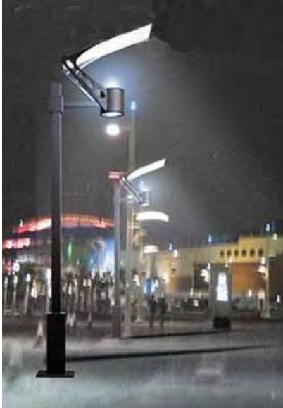
Figure I.2. Energy Efficient Technology. LEDs generate a lot of light with little electricity. Reflectors accompany LEDs to illuminate larger areas, and can be designed to be compatible with traditional light fixtures.
