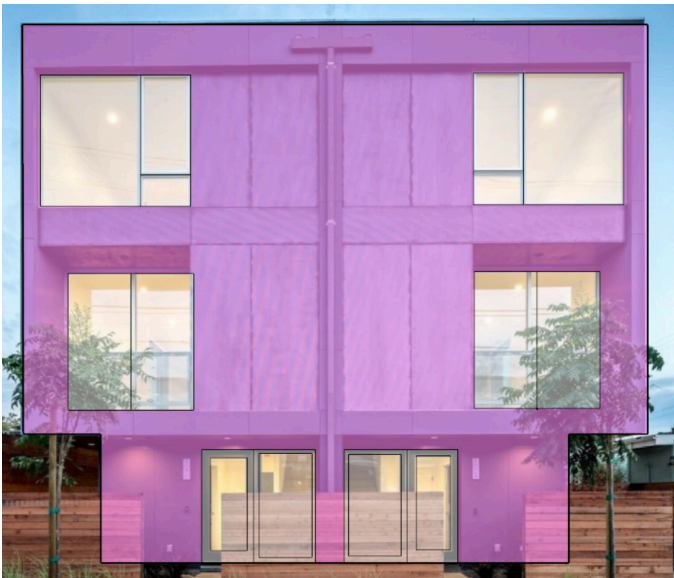
1030 Grayson, Berkeley Openings are approximately 32%
