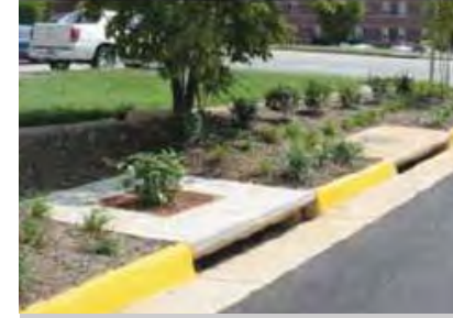
Figure g.6. Tree Basins. Bio-retention features can accompany new trees, but special engineering and tree survival concerns must be addressed.
