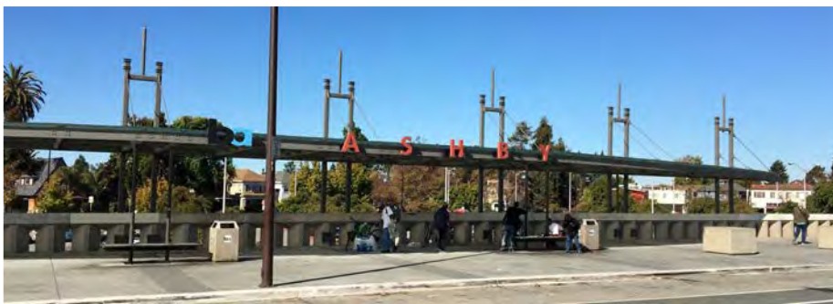
The Ashby BART Station
