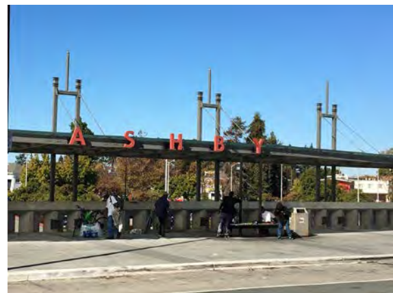
The Ashby BART Station
