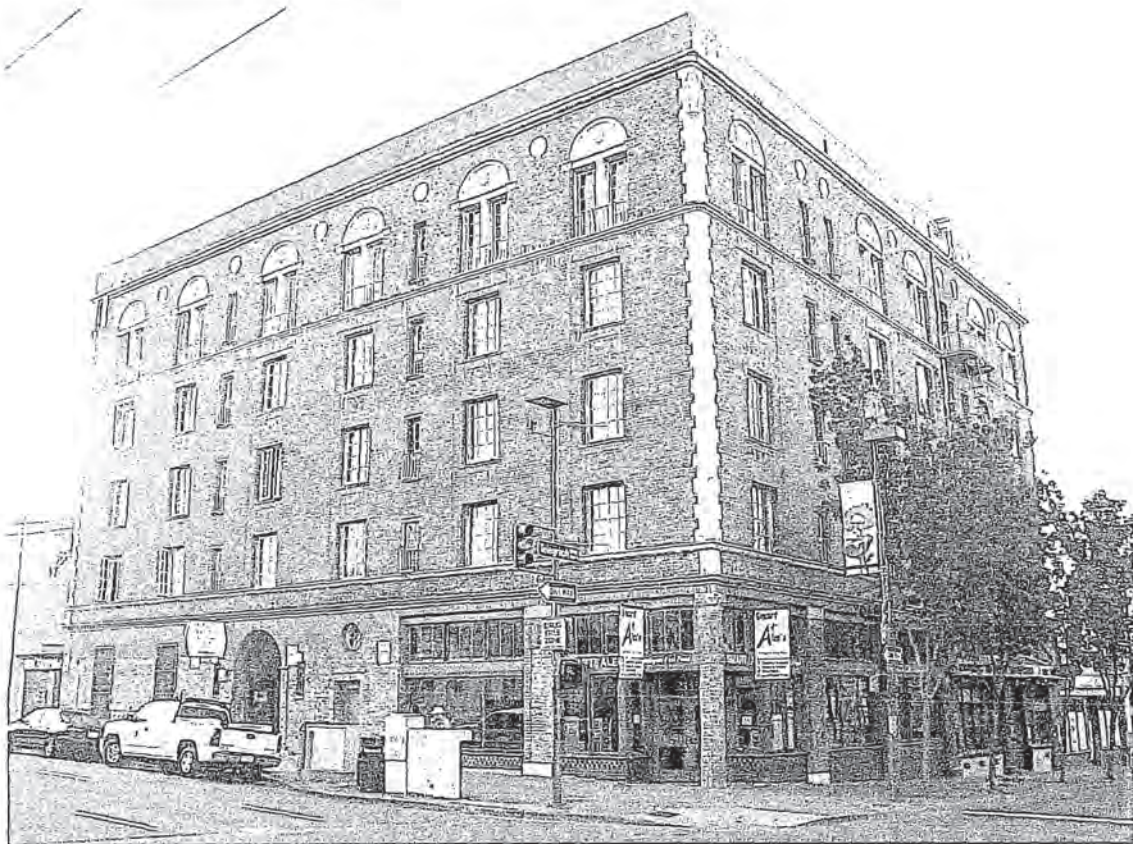
Photo 1. August 2007. The Cambridge Apartments, looking southeast.
