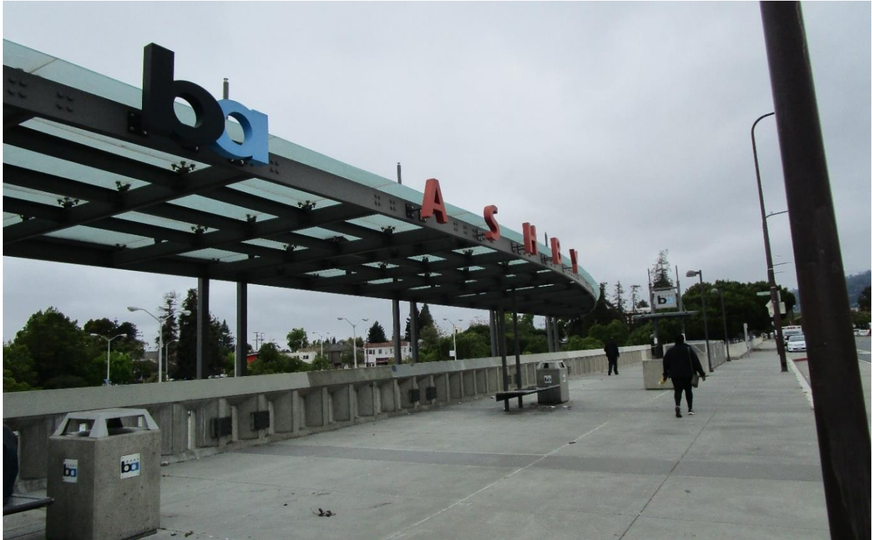
Figure 16 Ashby BART Station, Street-Level Deck along West Side of Adeline Street, Featuring Non-Original Canopy and Signage, Facing Northwest
