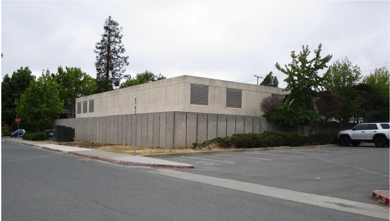
Figure 12 Utility Building at the North Berkeley BART Station, South and East Elevations, Facing Northwest
