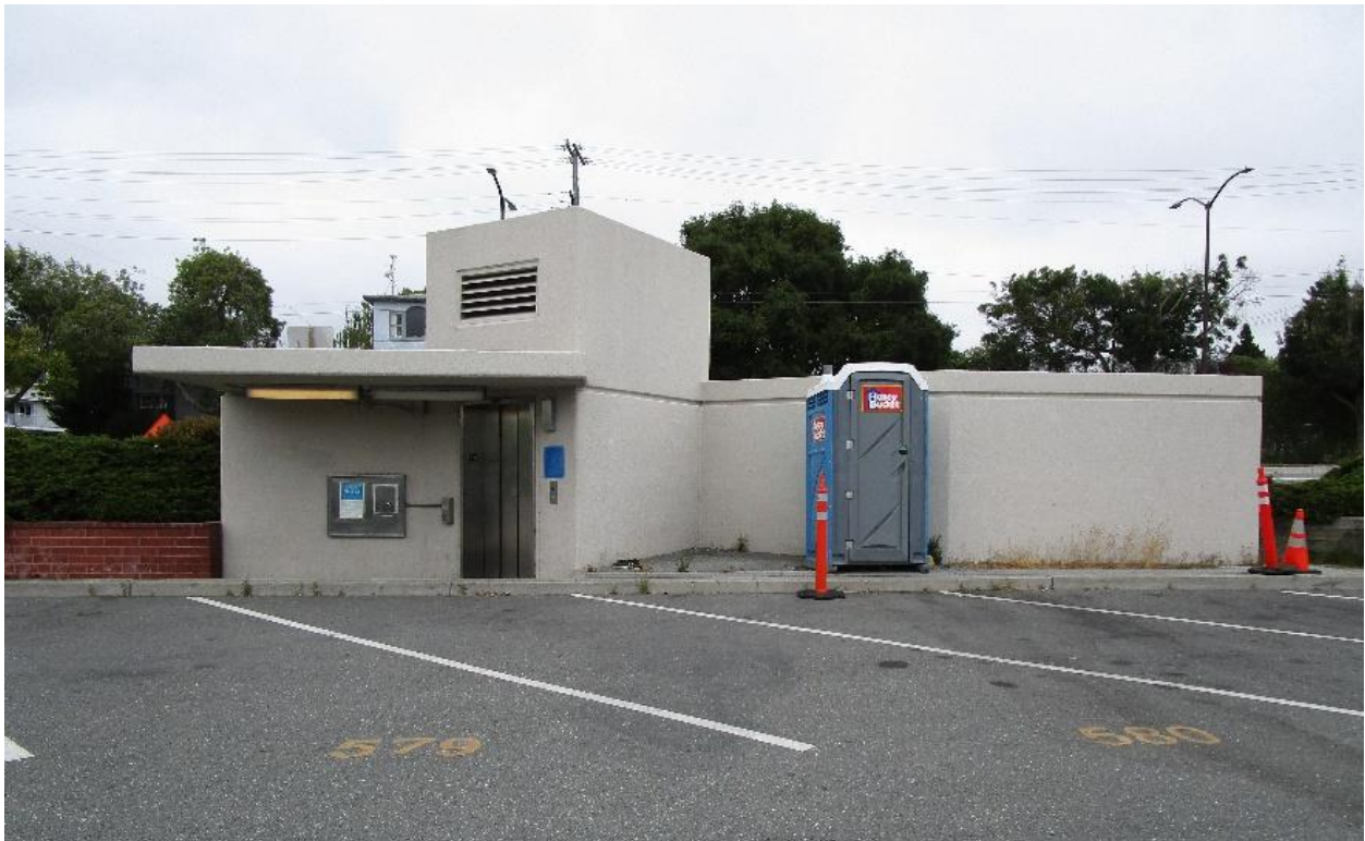
Figure 13 North Berkeley BART Station Elevator Shaft, West Elevation, Facing East
