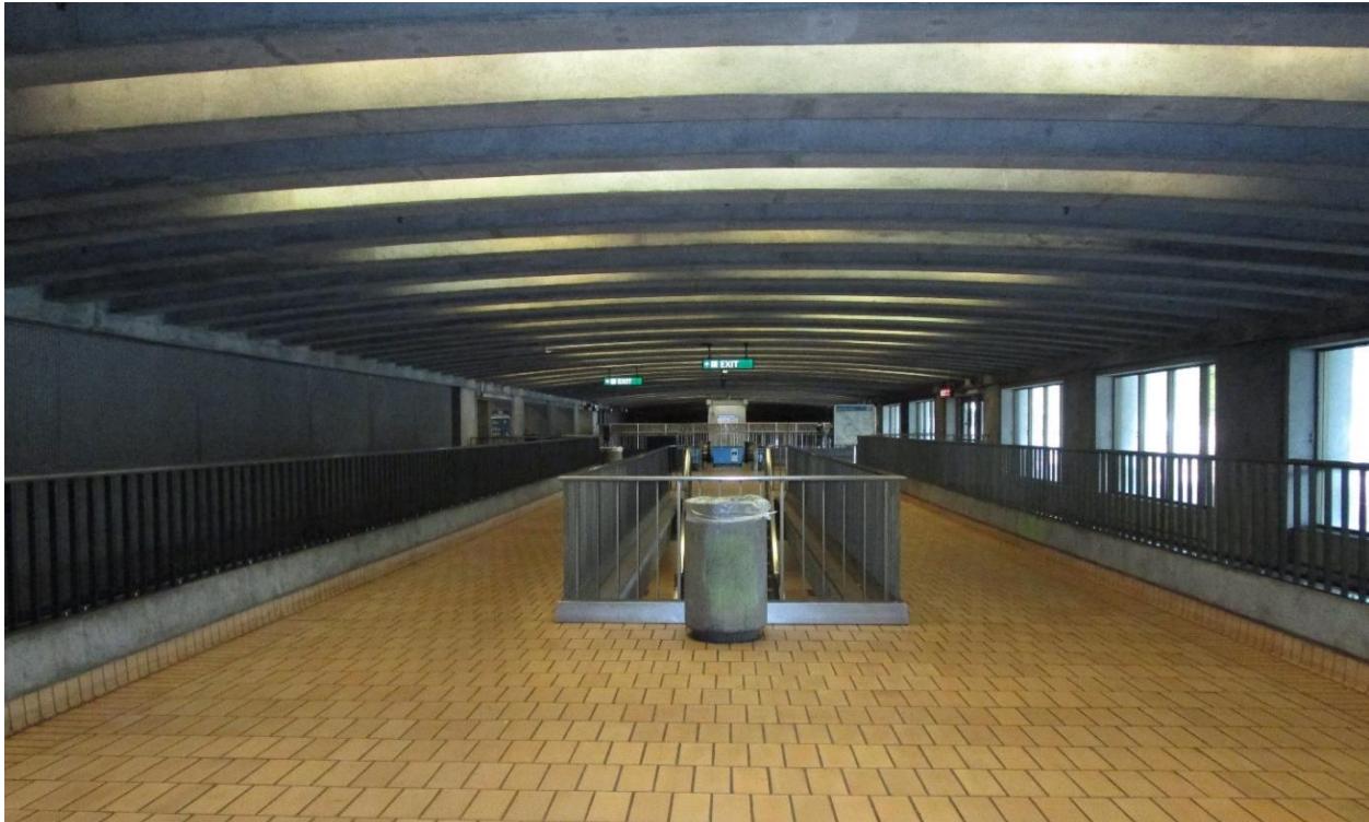
Figure 18 Interior View of Paid Area of the Ashby BART Station Concourse Level
