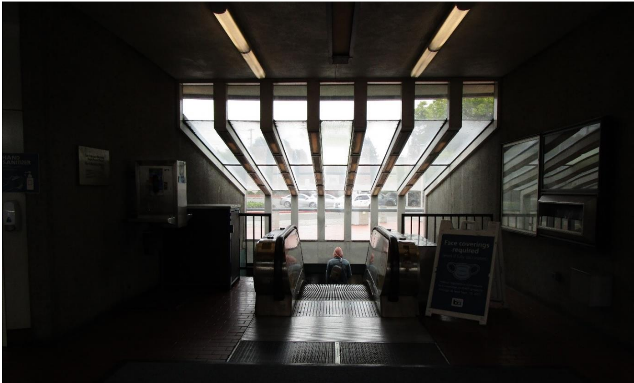
Figure 10 North Berkeley BART Station, Interior View of Skylight and Escalator from Concourse Level
