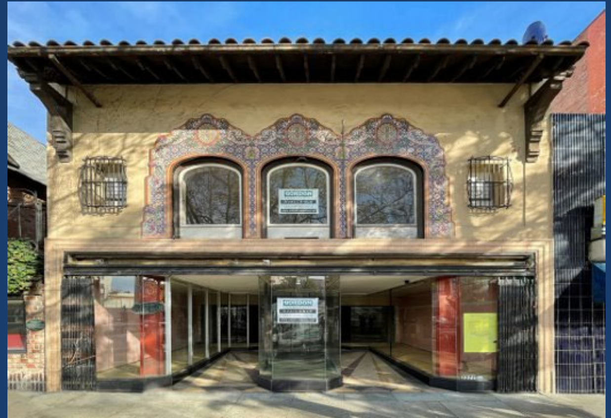
Commercial space with "For Lease" signs and an AUP application pending
