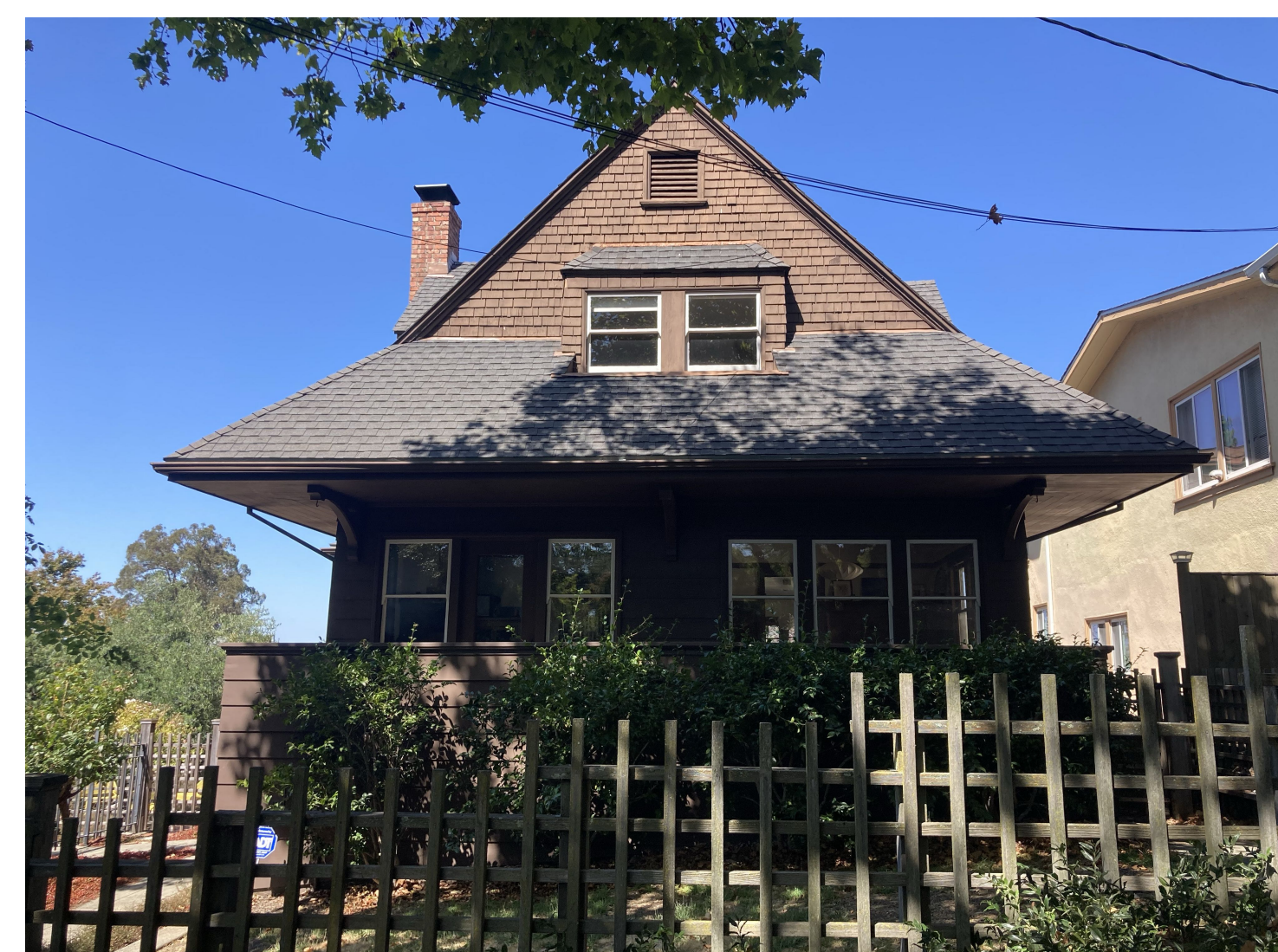
2. EXISTING HOUSE PHOTO - SOUTH ELEVATION
