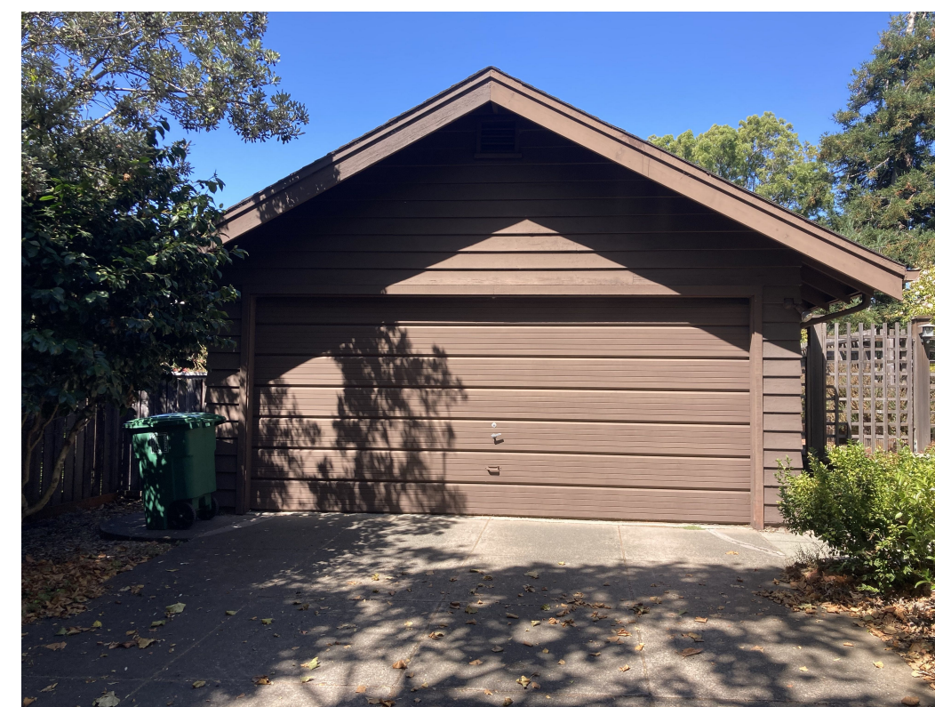
6. EXISTING GARAGE PHOTO - SOUTH ELEVATION
