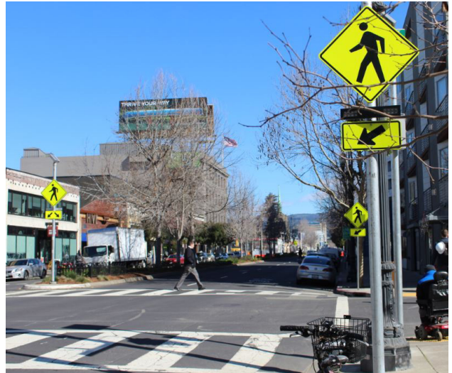
RRFBs (Broadway/23rd St, Oakland)
