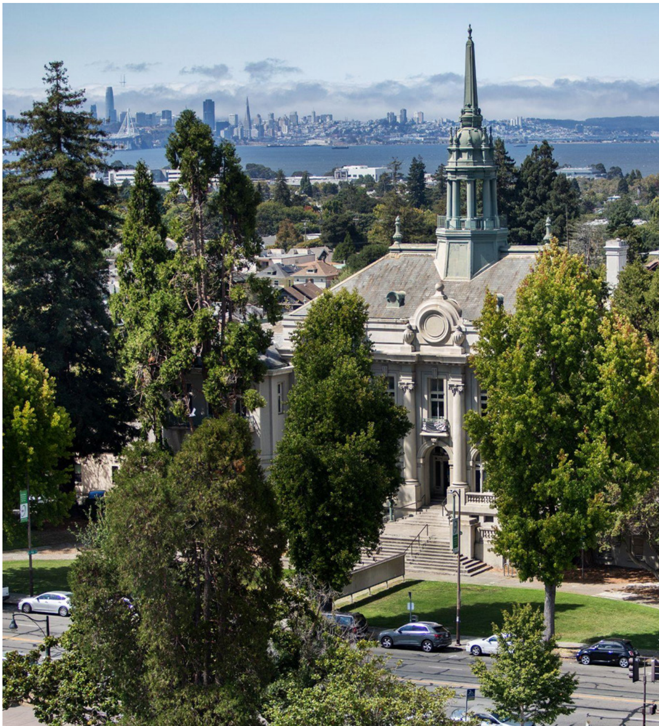
View to Maudelle Shirek Building from roof of Veterans Memorial Building
