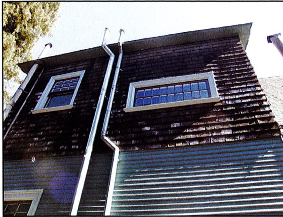
Fig. 4. The dormer on the north, showing the horizontal stair landing window. Daniella Thompson, 2021
