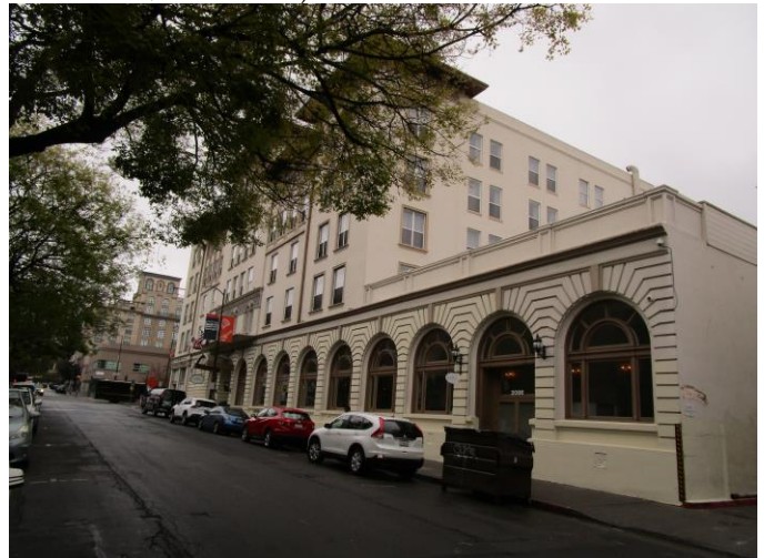
North elevation, view southeast. (Rincon Consultants, March 2022).
