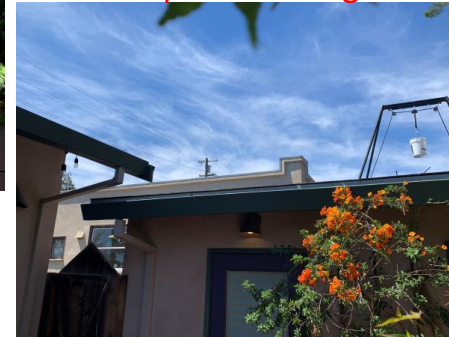
B – from patio looking north
