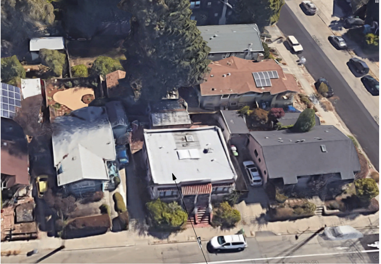
area of new addition
