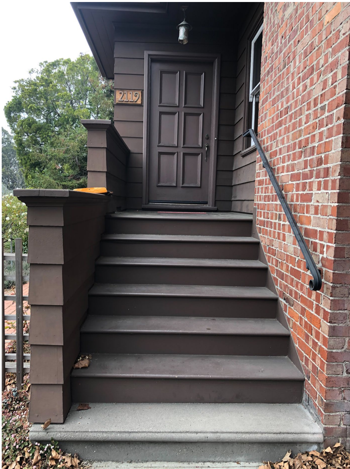
Fig.17 – 2119 Marin Ave. – West side entry
