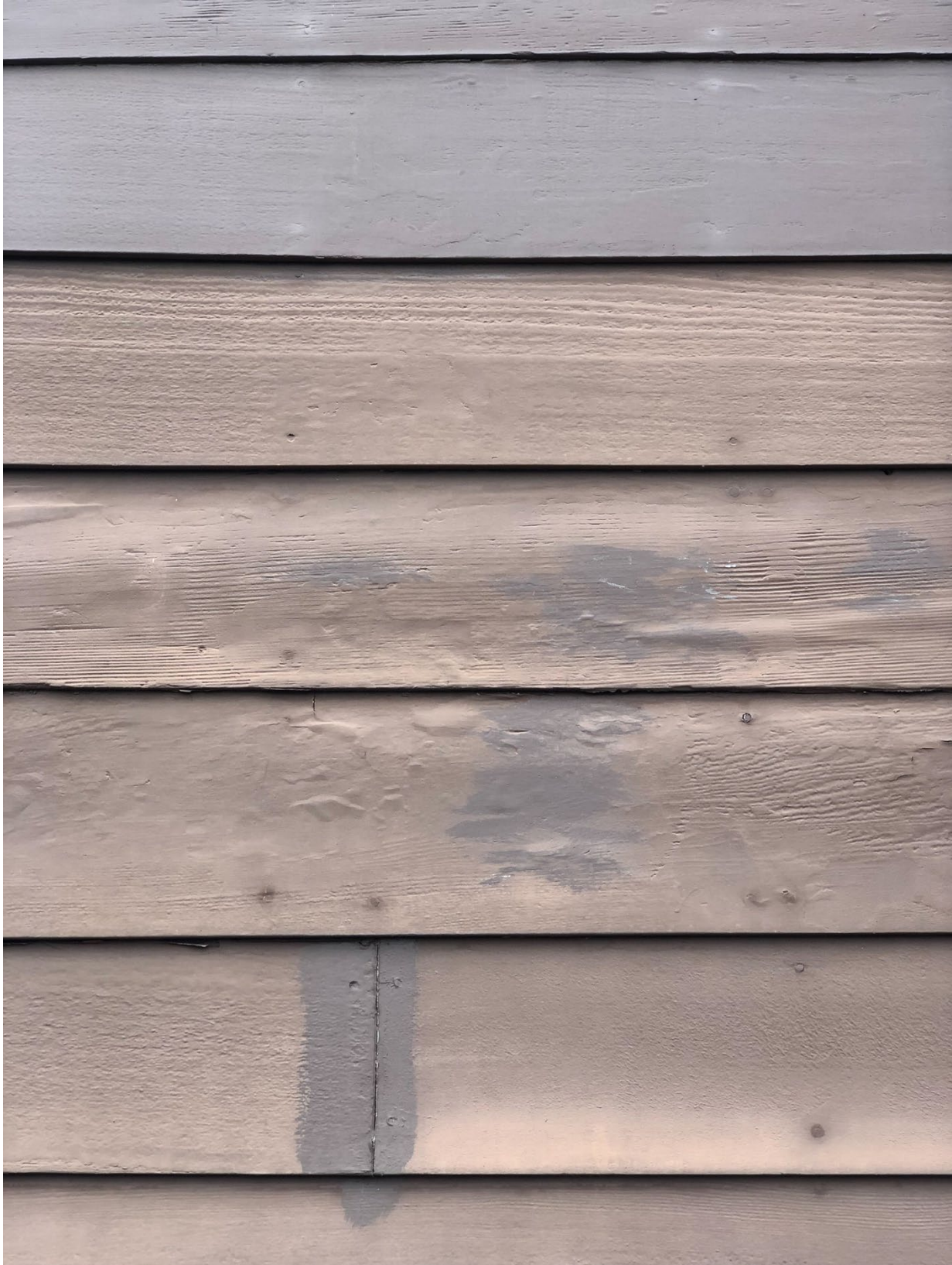
Fig.24 – 2119 Marin Ave. – Redwood siding
