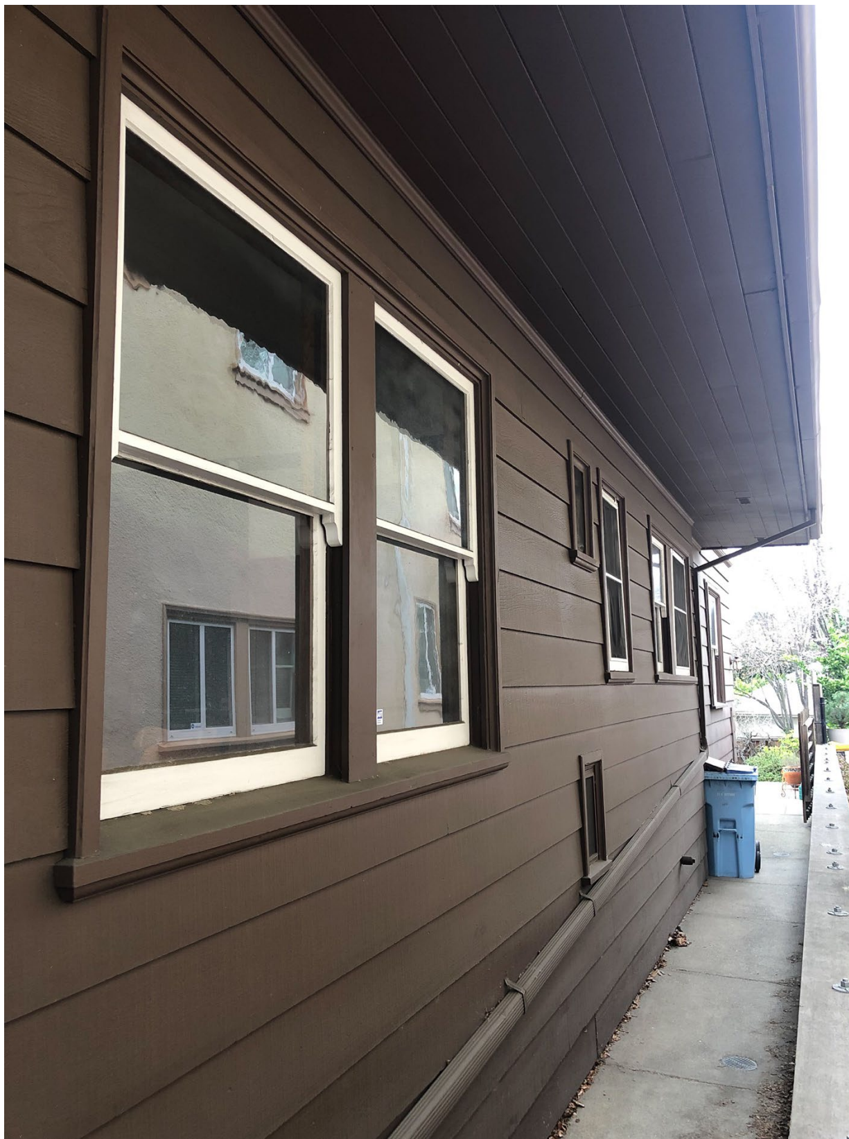
Fig.23 – 2119 Marin Ave. – East side
