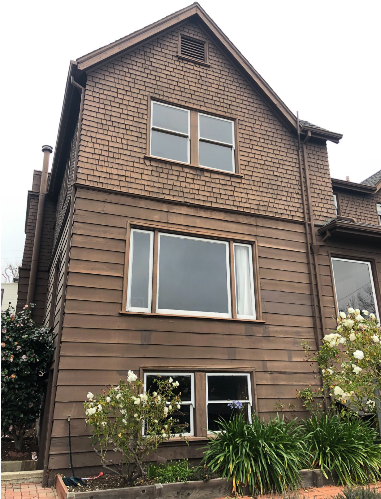
Fig.22 – 2119 Marin Ave. – West side, rear
