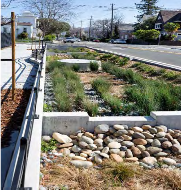
Green infrastructure installation at Woolsey Street
