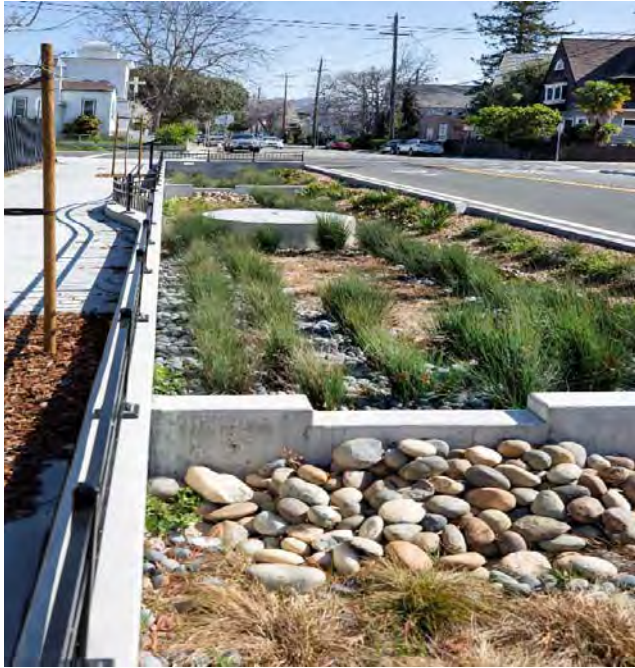
Green infrastructure installation at Woolsey Street
