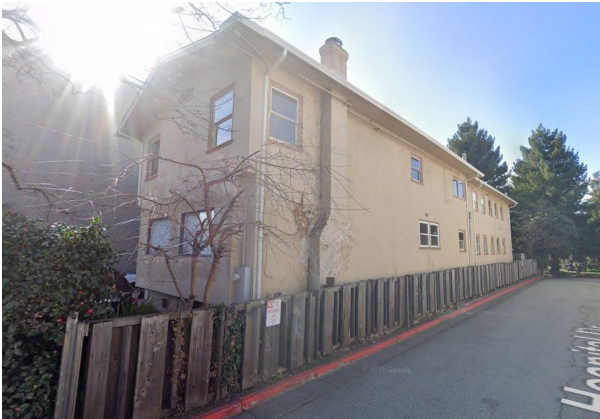
Conversion of care facility to duplex 3028 Regent Street 2 units
