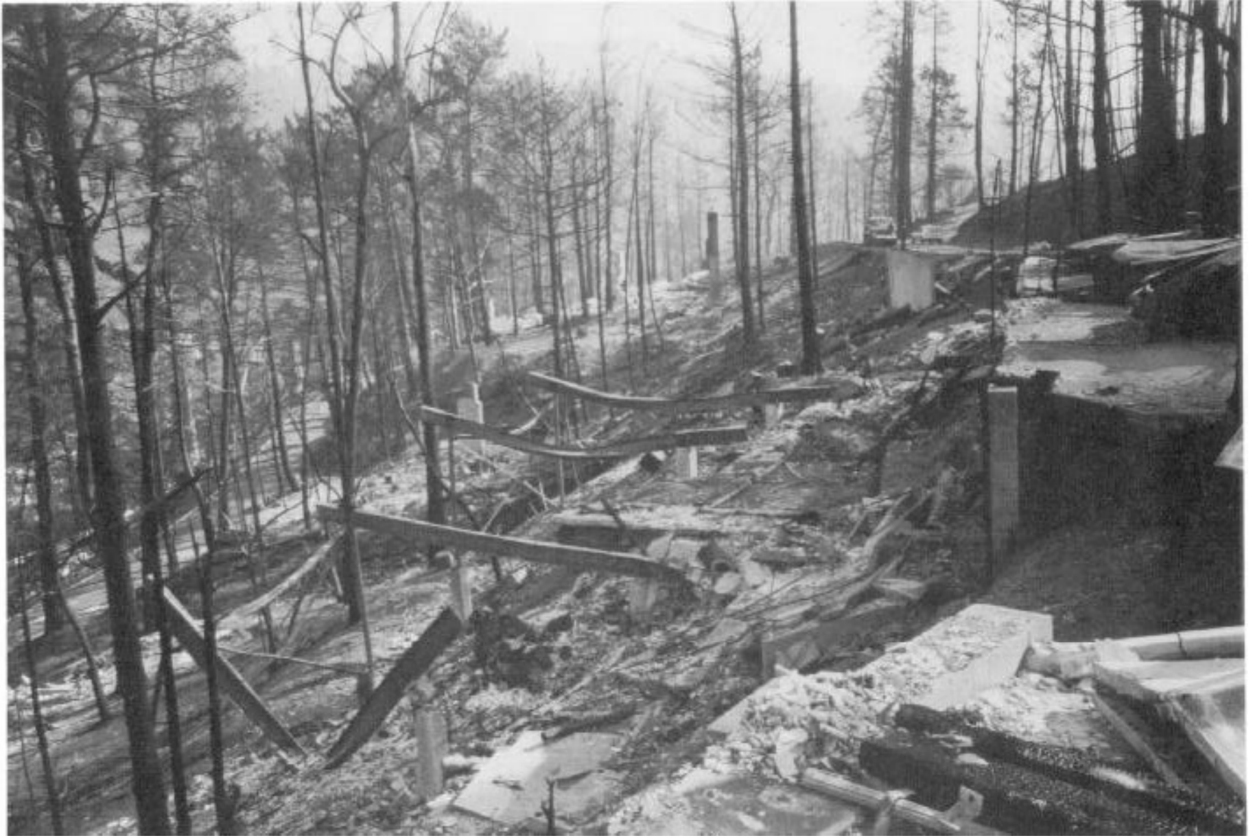
Buckled steel beams mark the location of a destroyed home on Buckingham Boulevard.
