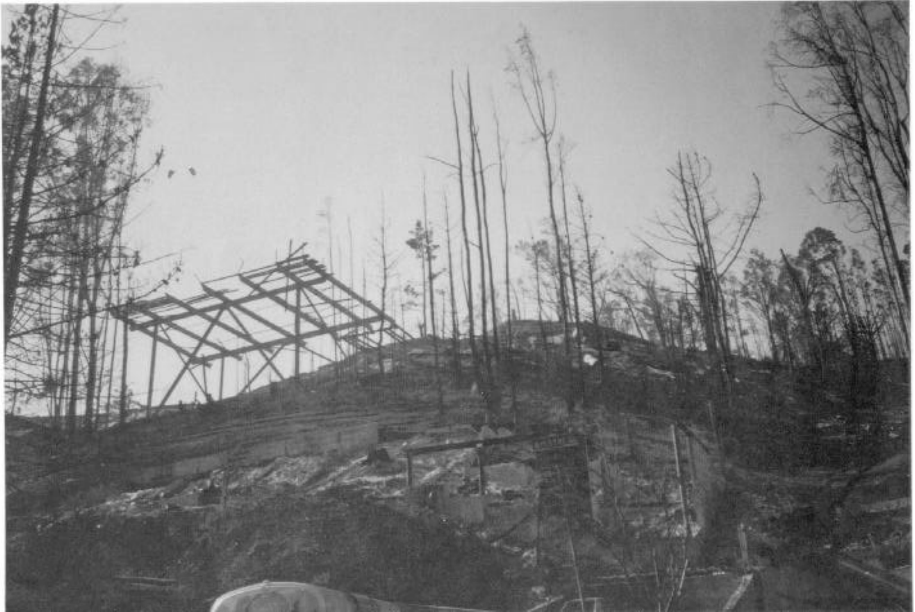
All that remains of one hillside home is the steel supporting structure for the main floor.
