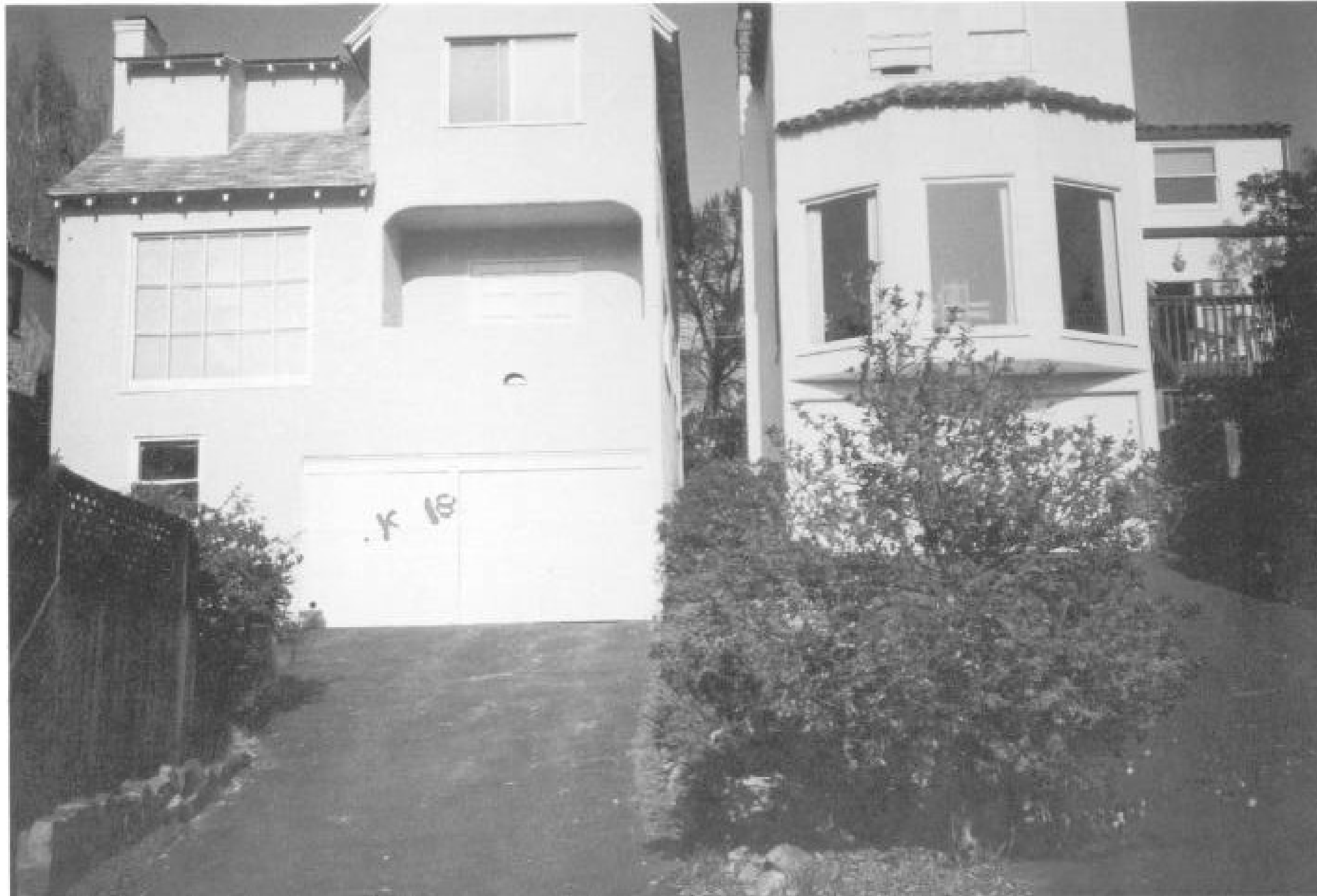
Typical homes on western edge of fire area.
