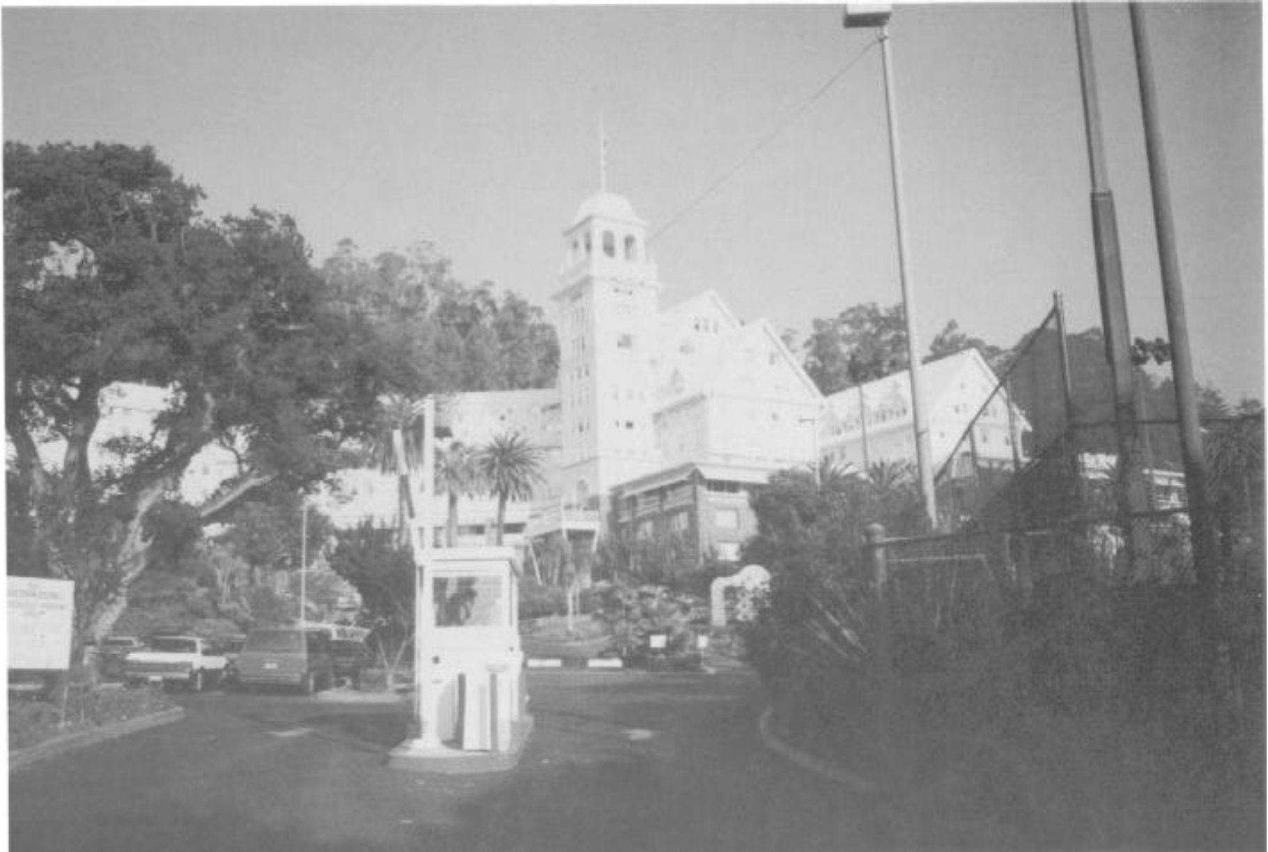
The Claremont Hotel - 5 - story wood frame structure in the path of the fire, considered a “conflagration breeder.”
