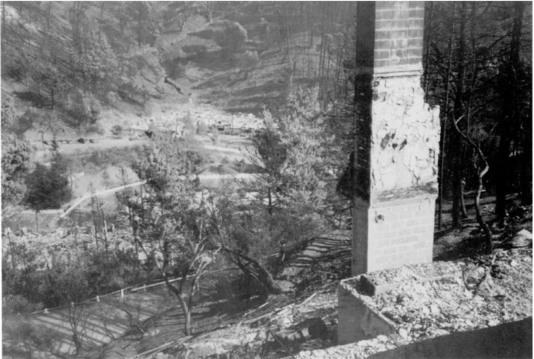
Looking down on the ruins of the Parkwood Apartments from Buckingham Boulevard. Tunnel Road is visible in the lower left corner.
