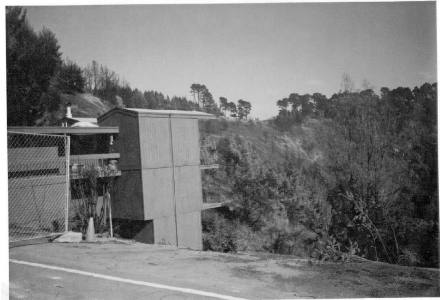
One of the few homes on Marlborough Terrace that was not destroyed by the fire. Houses on both sides burned to the ground.
