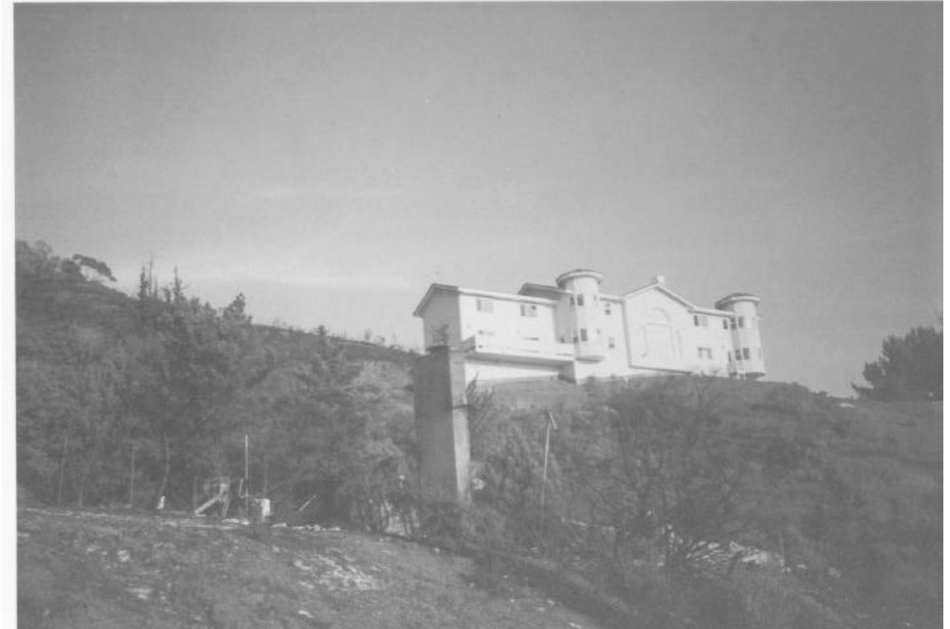
Large home saved by clear area around structure.
