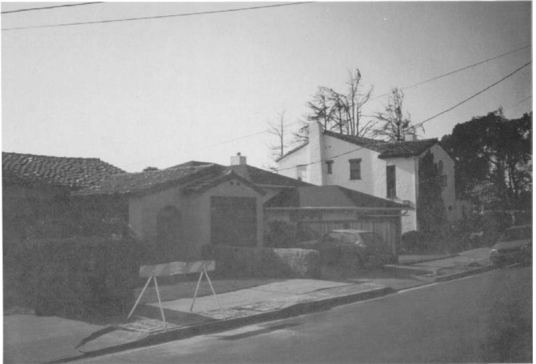
Homes saved within fire area - note non-combustible roofs.
