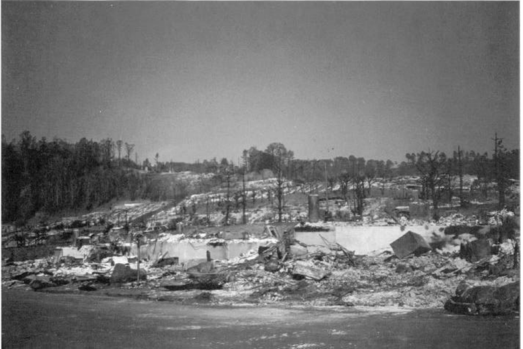
Total destruction of Hiller Highlands complex.
