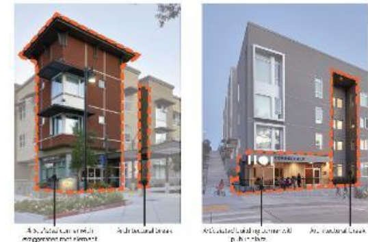
Fig. 3.1.2 Define context and building form at street level through architectural details such as cornices, massing, and recessed entrances that distinguish buildings from one another.
