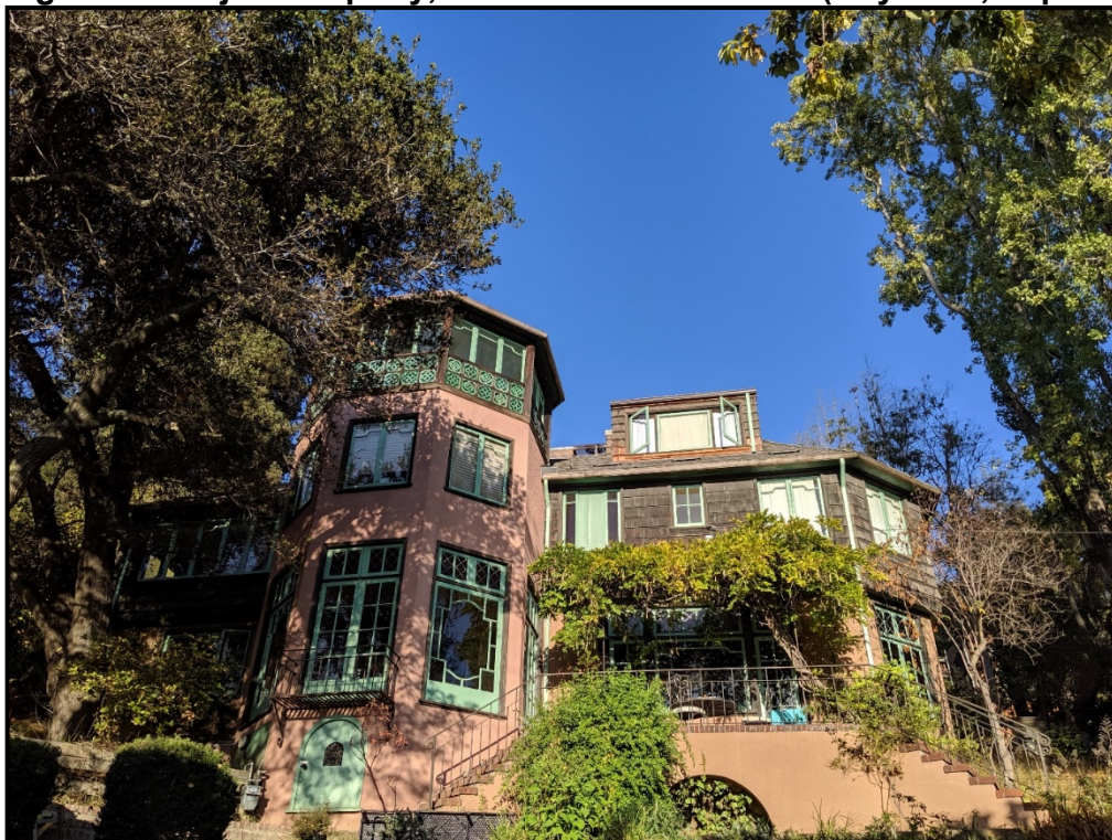
Figure 2: Subject Property, current site conditions (City Staff, September 2020)
