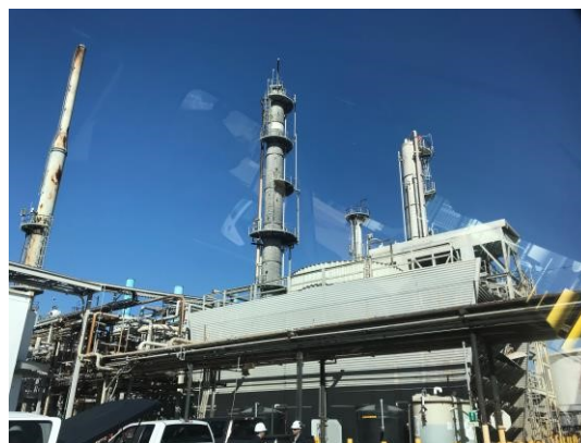
Figure 4. World Energy’s Paramount plant (photo by GNA)
