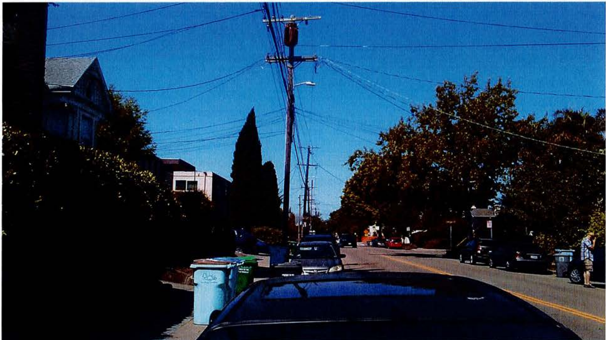
Photo 1: Taken from Dwight Way facing West near Jefferson Avenue with poles and overhead utilities
