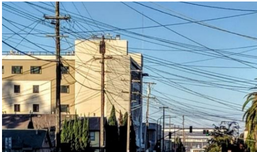
Dangerous overhead wires
